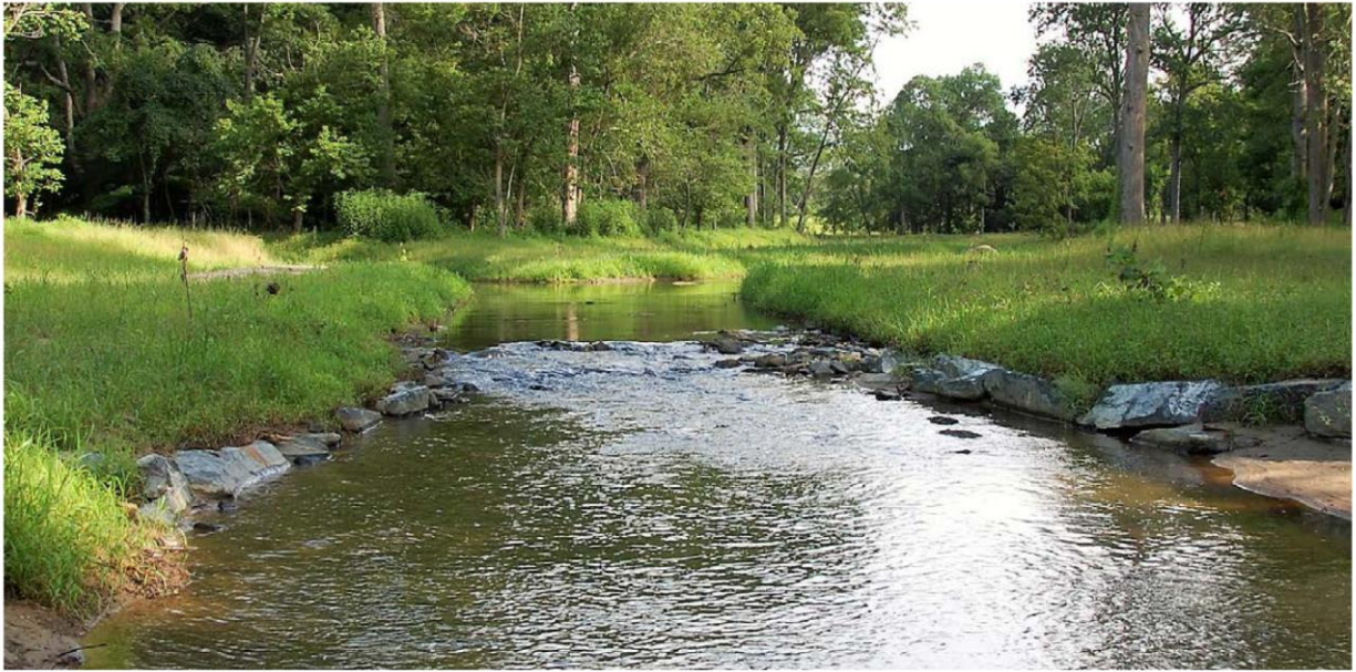
Figure 1. Cross vane on Upper Little Patuxent River, Maryland used to protect a sewer line which crosses the channel just upstream of the vane. (photo courtesy of Johnson, Mirmiran & Thompson, Inc.).
