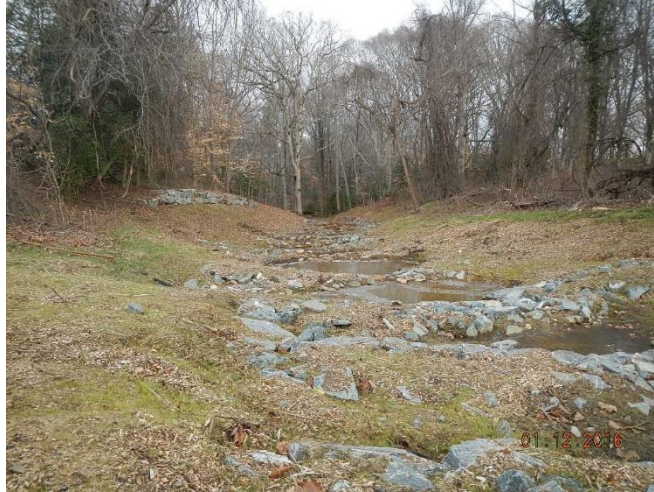
Figure 2.12: Eastern Tributary SPSC in Annapolis, MD several years after its 2013 construction. Photo by Tess Thompson (2016), used with permission.
