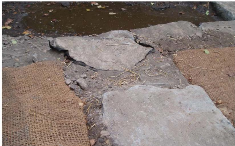
Figure 5. Vane rocks should fit snugly together and be chinked with smaller rock with a wide range of sizes. (Design by Wetland Studies and Solutions, Inc.)
