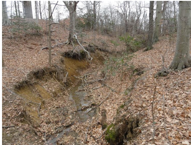
Figure 2.11: Eastern Tributary site in Annapolis, MD before SPSC construction. Photo by Terry Schuman with Bay Engineering, Inc. (2011), used with permission.
