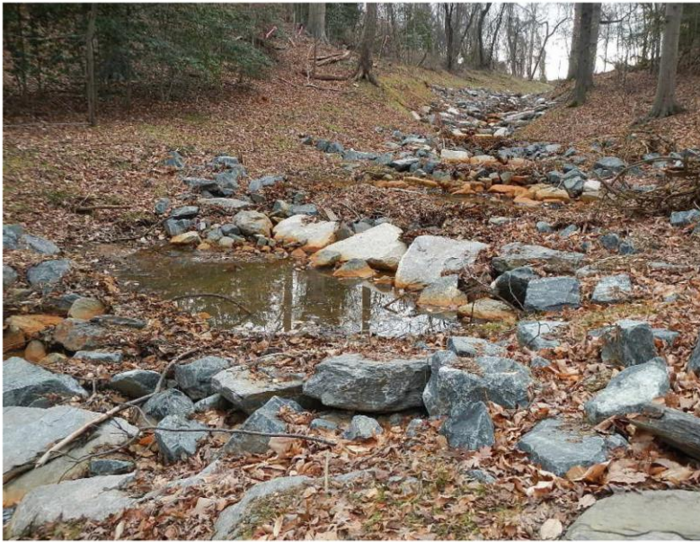
Figure 2. Regenerative step pool conveyance directs runoff from parking lots to Broad Creek, Annapolis, MD.
