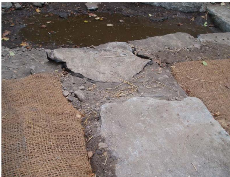
Figure 3. Rocks should fit snugly together and be chinked with smaller rock with a wide range of sizes. (Design by Wetland Studies and Solutions, Inc.)
