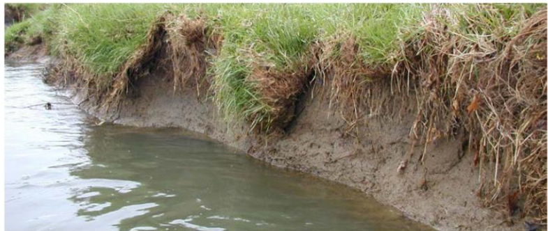
Figure 1. Single-arm vanes redirect flows from banks, reducing erosion caused by high flows.
