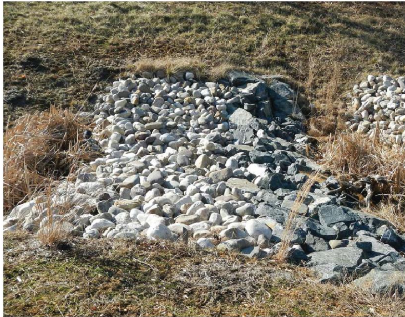
Figure 3. Regenerative step pool conveyance weirs have a cobble apron on the upstream side, reinforced with boulders.
