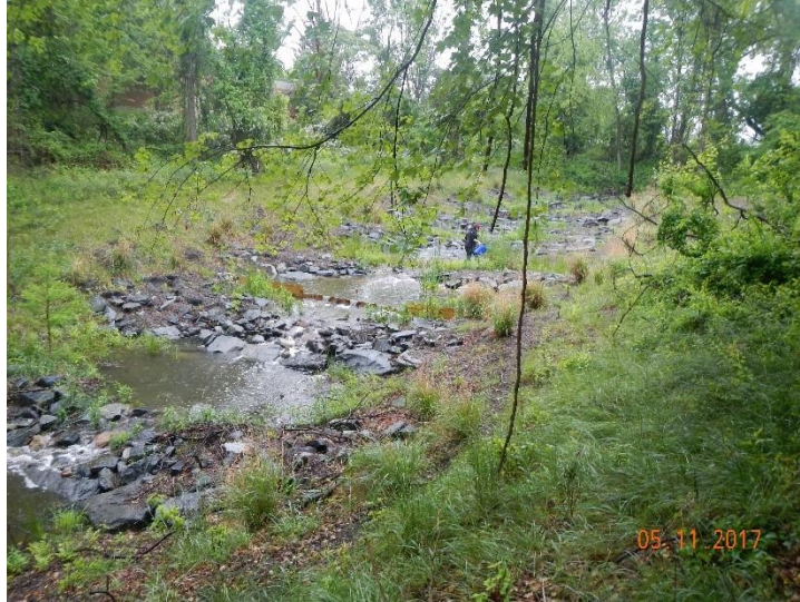
Figure 4.3: Eastern Tributary SPSC with upstream compound weir during the May 11, 2017 controlled flow releases. Photo by Tess Thompson (2017), used with permission.
