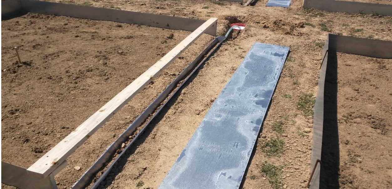
Fig. 4-3. The gutter, hose and bucket runoff collection section. The gutter was then covered by the steel plate on the right to prevent rainfall from directly entering the gutter.
