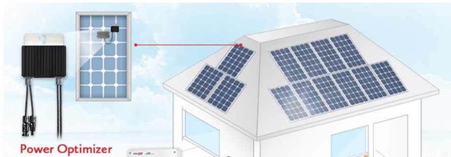
Figure 5.2. PV modules and power optimizers are installed on the roof.
