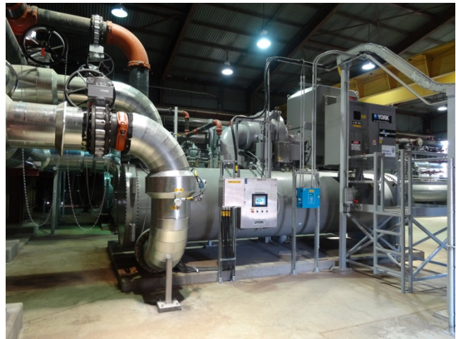
Fig. 12. Glycol/water chiller in plant room
