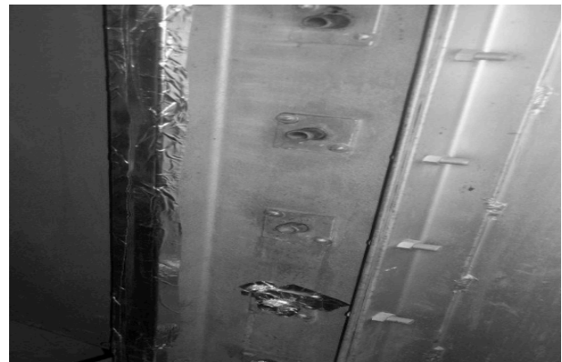
Figure 4. Louvers holes on the duct surface
