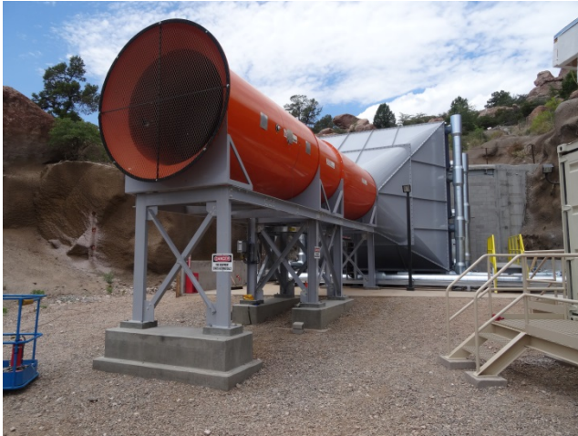
Fig. 9. Surface cooling coil and force fan
