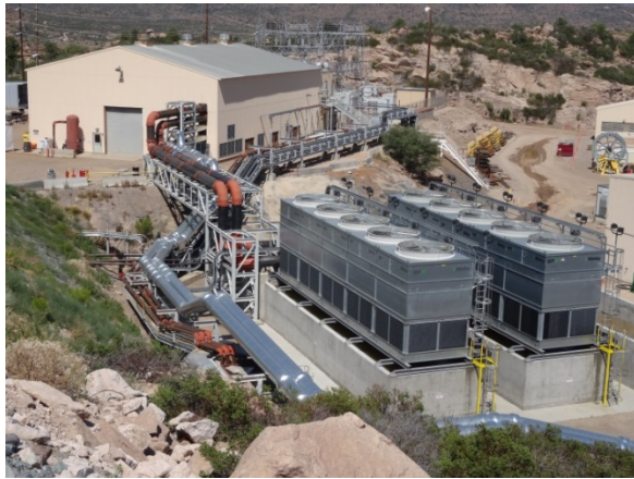
Fig. 13. Plant room, condenser cooling towers and insulated piping
