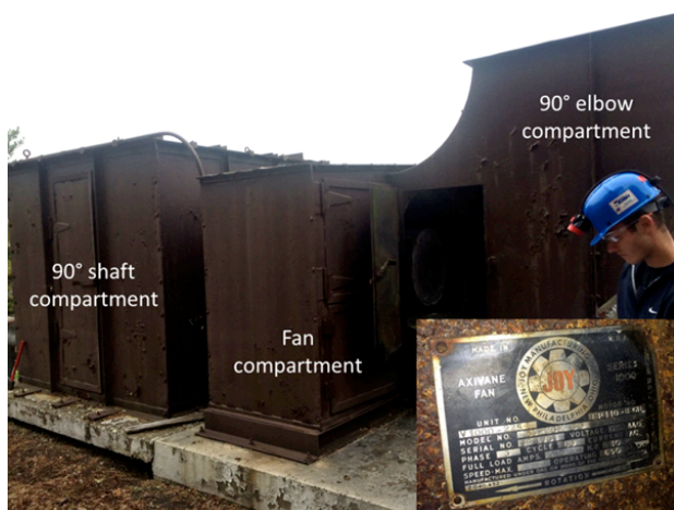
Fig. 3. Three components of the SRCM fan structure.
