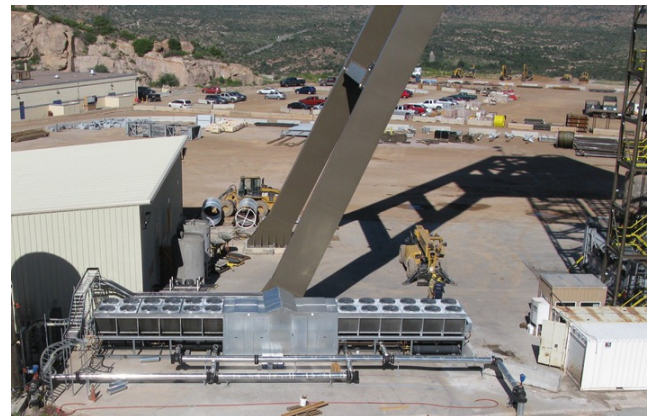
Fig. 2. Air cooled refrigeration machines
