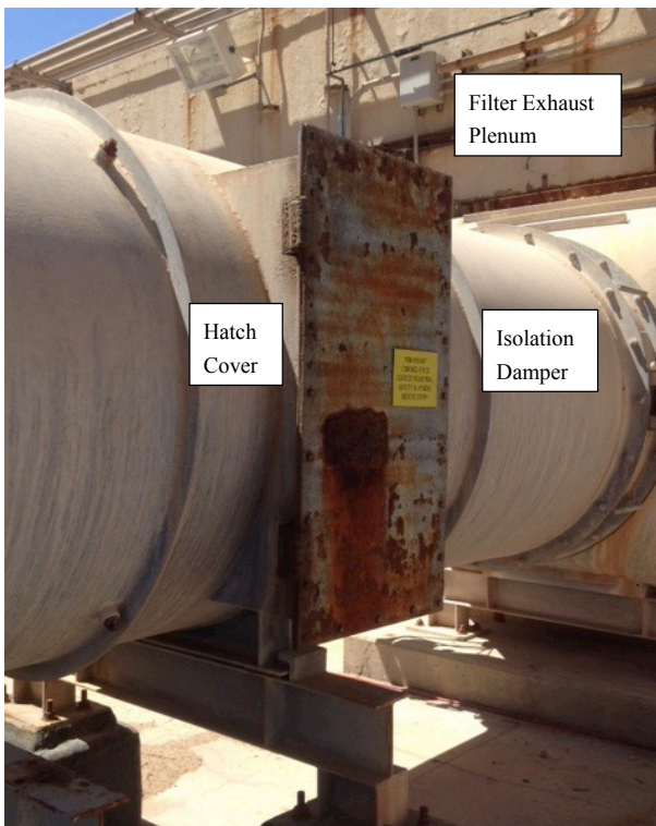
Fig. 8. 860 fan access hatch with isolation damper.
