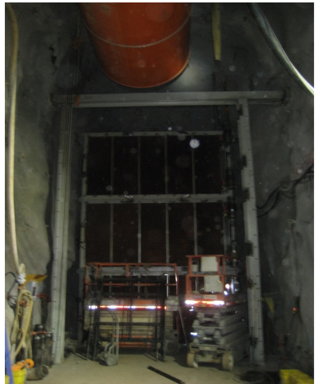
Fig. 11. Pump Level cooling coil under construction
