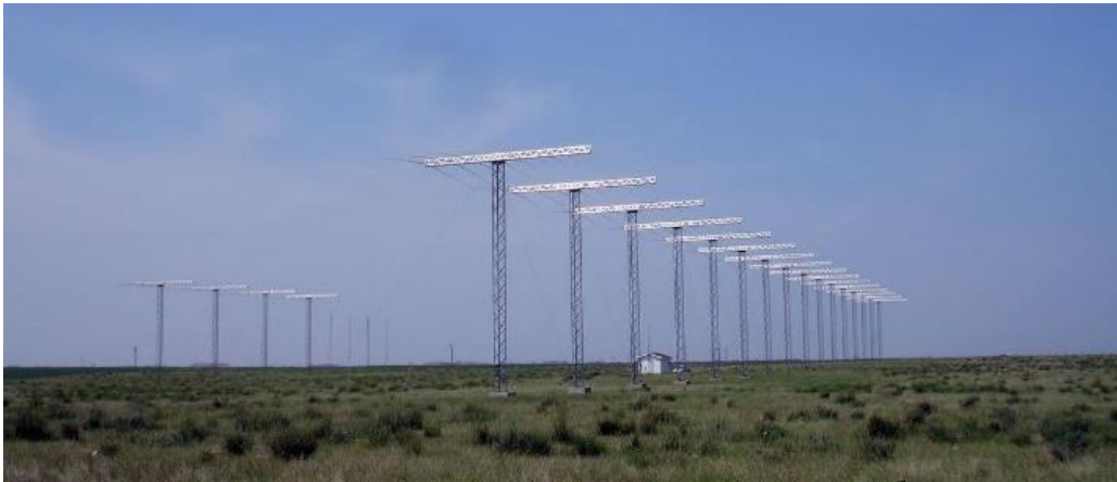
Figure 1.3. SuperDARN Antenna Array in Holmwood SDA, Saskatoon [6]
