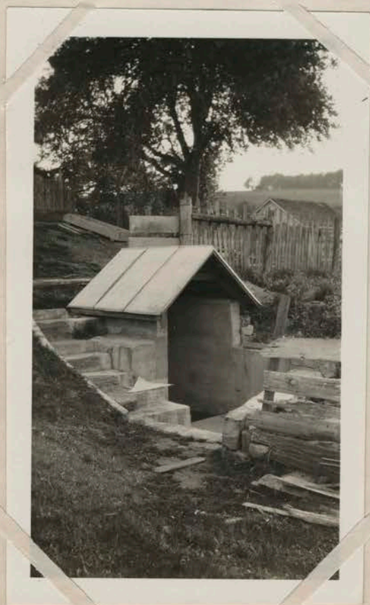
A Spring made safe from Pollution by concrete. Rockingham County. Sanitation Project.
