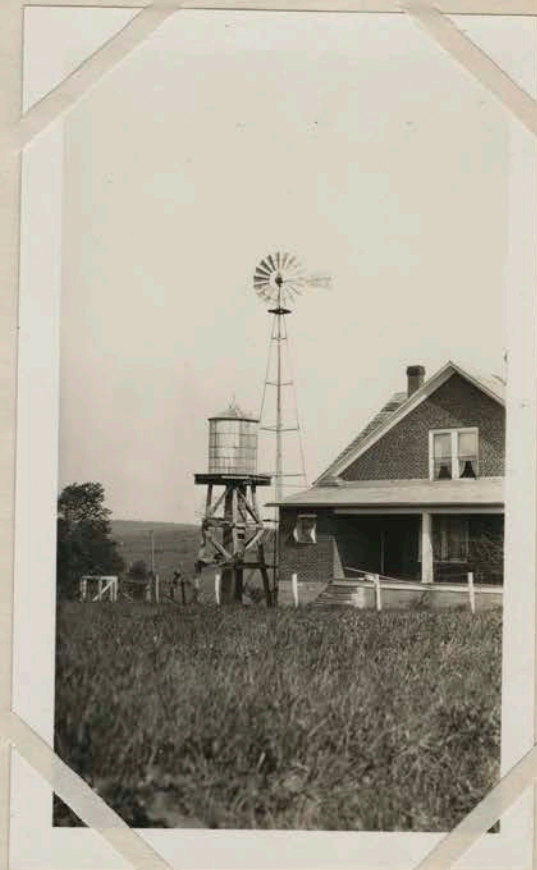
The windmill and Gravity Tank are Great labor Savers and make a satisfactory Farm Water system.
