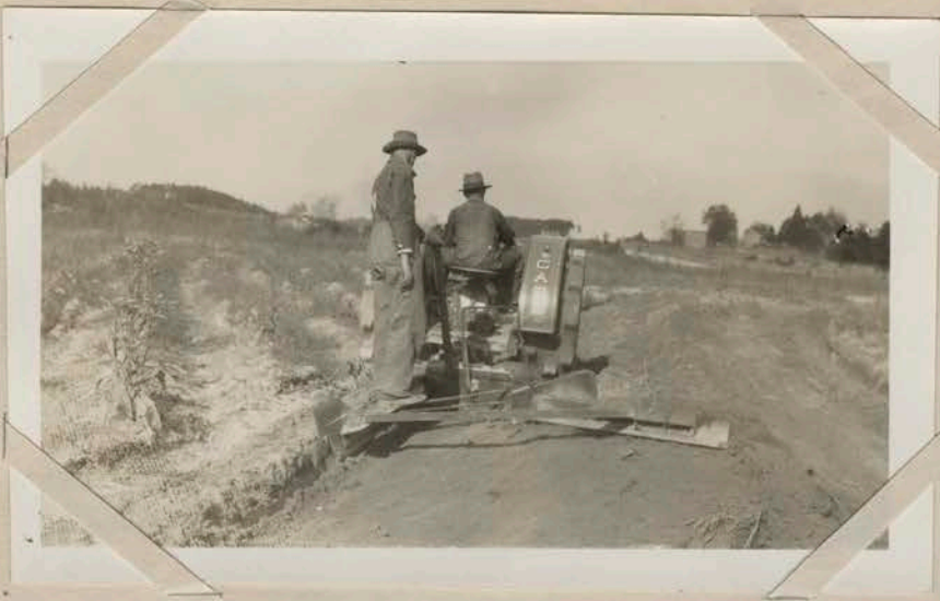
Constructing Terrace with Tractor and Steel Grader Halifax County.
