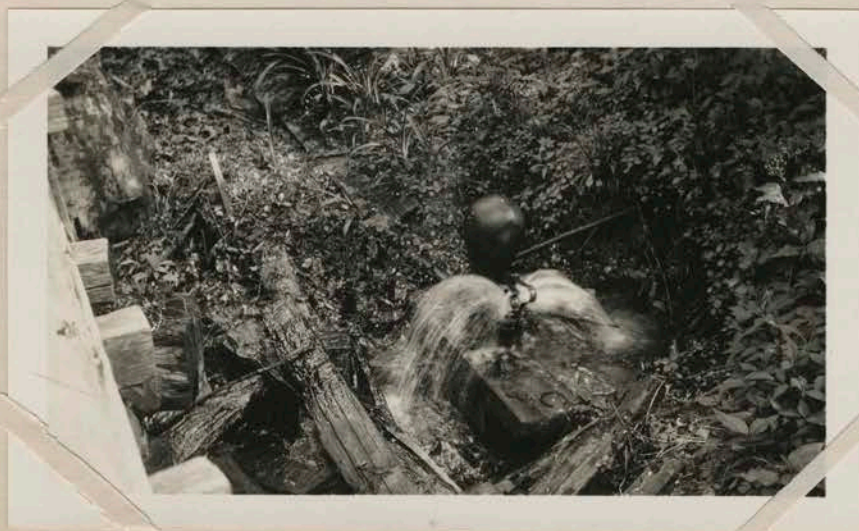
The Ram Is Ideal For Pumping Water On The Farm. Rockingham County. Water Supply Project.
