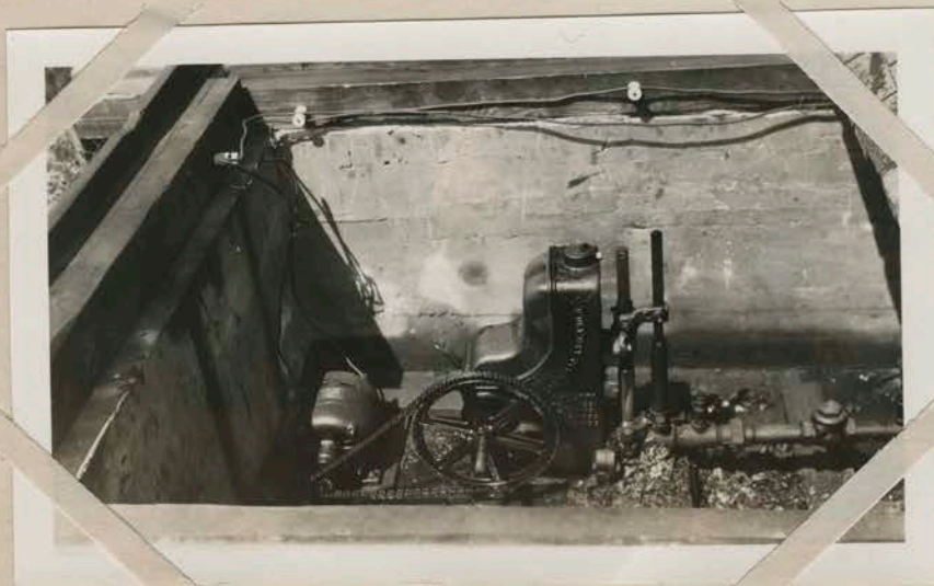
Motor Driven Pump. Pittsylvania County.
