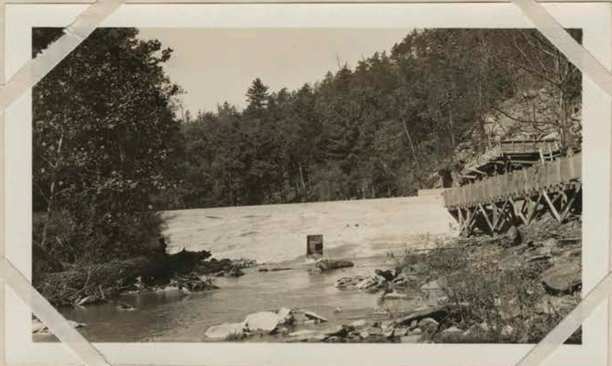
Wood Flume to convey the water to Power Plant.
