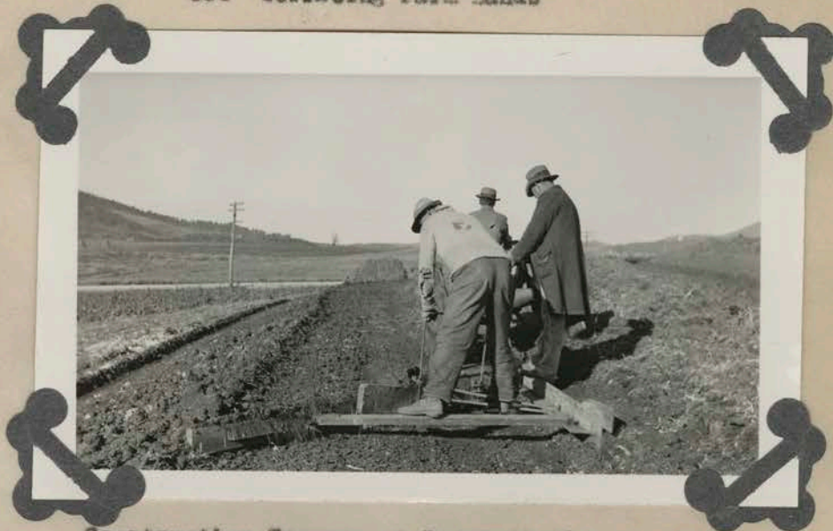
Constructing Terrace at Demonstration on Farm in Botetourt County
