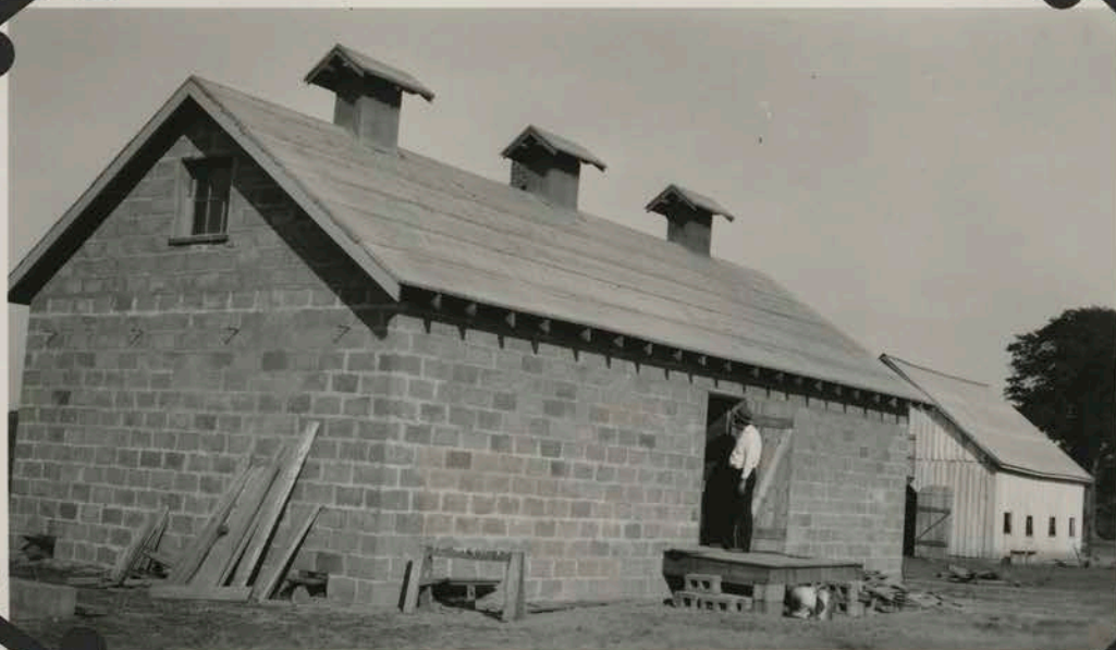
Cinder Block Sweet Potato Storage House in Princess Anne County (2,000 bushels) built from our plans which is proving satisfactory. There are now 43 individual houses in this county.
