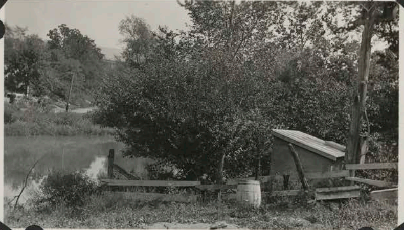
Pump House at Creek, Turkey Knob Orchard Water Supply
