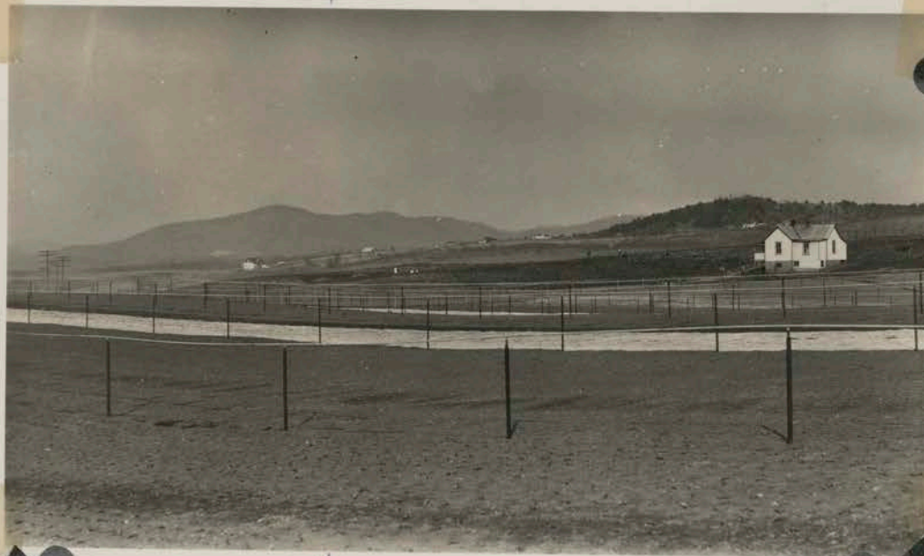
7. A General View of Part of the Sanderson Overhead Irrigation Project
