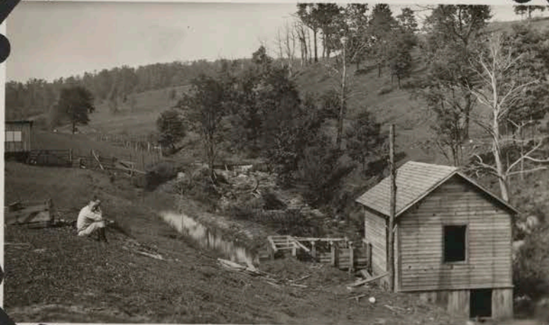
Dam, head race and power house. Farm water power project in Floyd Co. that furnishes lights for farm house and buildings.
