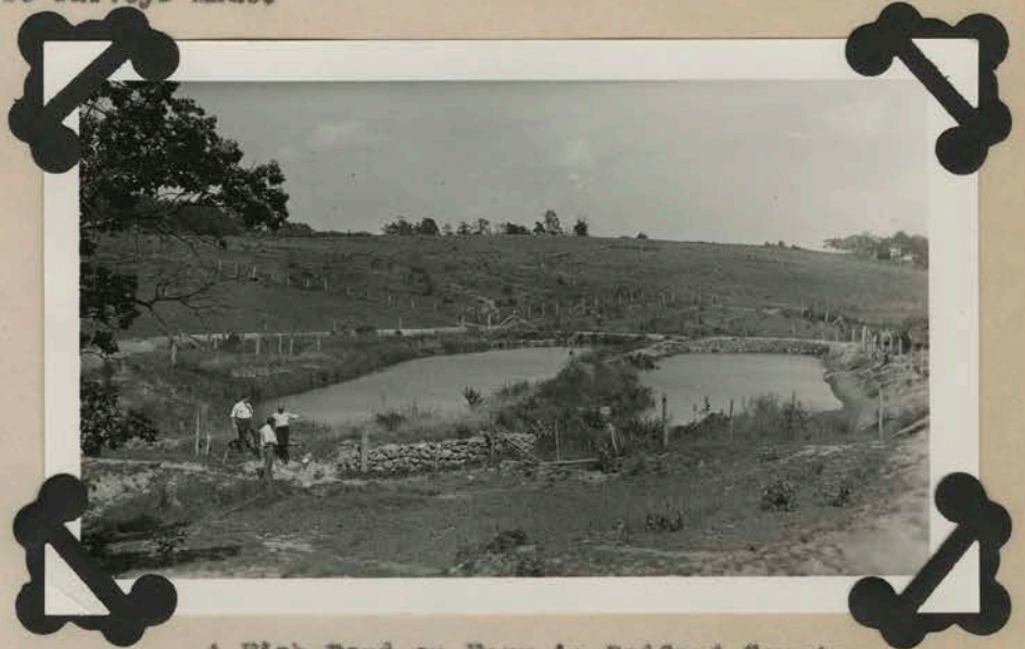
A Fish Pond on Farm in Bedford County
