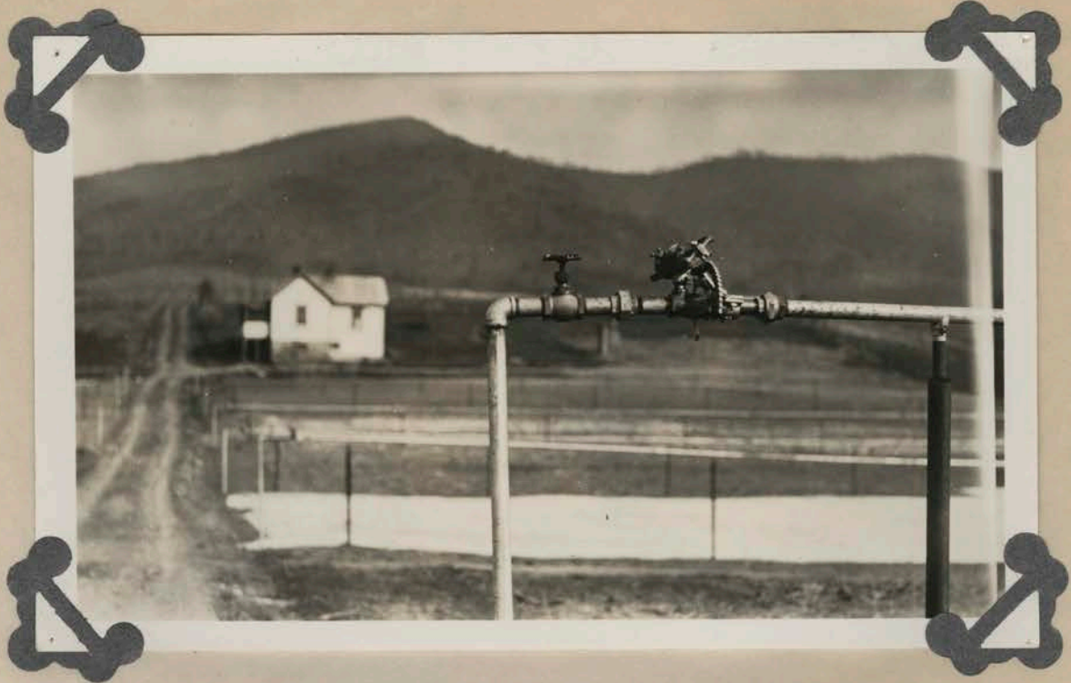
5. Automatic Oscillators Turn Sprinkler Pipes From Side to Side so that Water is Evenly Distributed on Both Sides of Line
