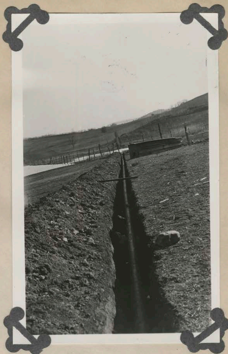
3.- 5" Second-Hand Boiler Tubing Was Used on All Mains Which Resulted In Considerable Saving
