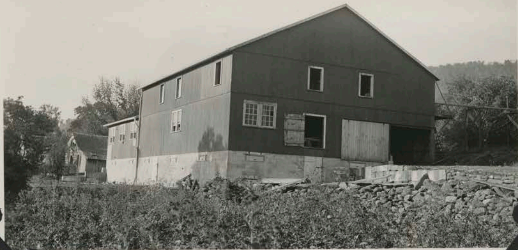
Apple Common Storage House, (11,000 bushels) - Franklin County. Built from our plans. The design of this house is based on three years study of apple storage requirements.
