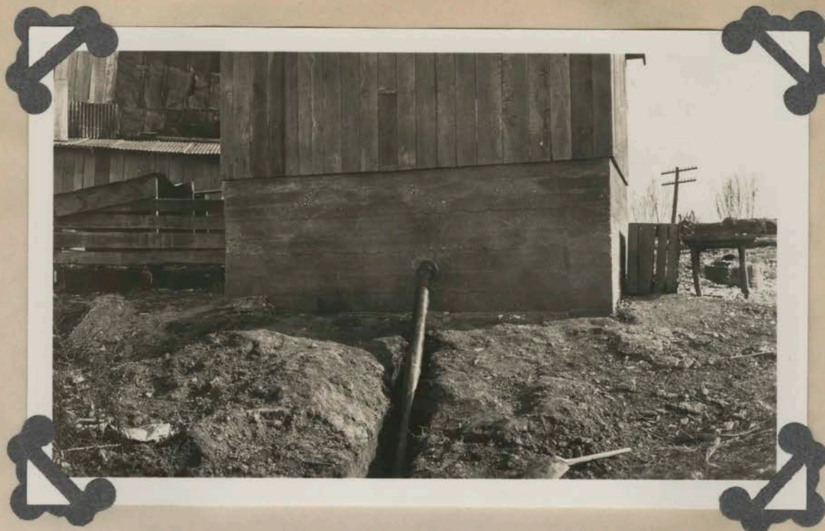
1. Rear View of pump House Showing Intake Pipe From Stream to Pump House
