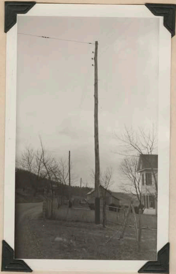
Farm line construction. Water power plant.
