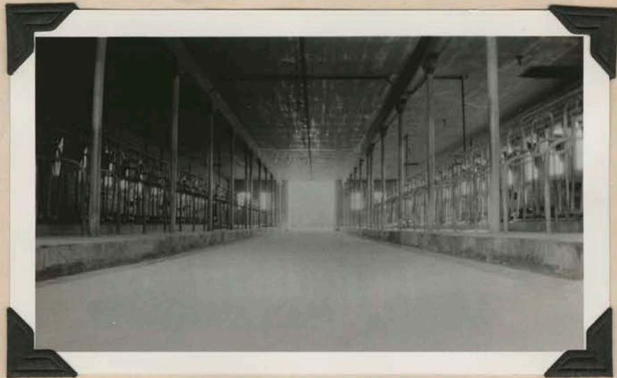
#16 - Interior view of 60 cow dairy barn.
