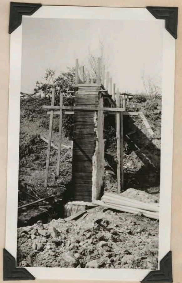
Turbine job in Patrick county.
