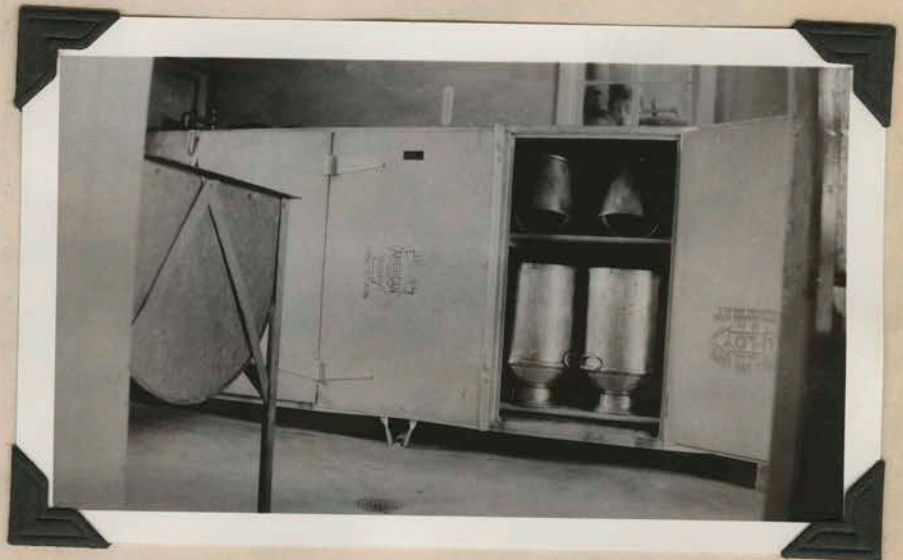
#12 - Interior view of #11 showing wash tanks and steam sterilizing cabinet required of all Washington shippers.
