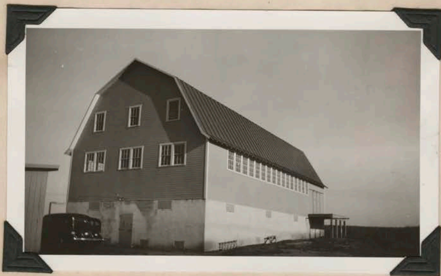
#2 - 40' x 80' combination apple packing and common storage for apples. V. P. I. Experimental orchards. Note ample lighting in middle of packing floor and ventilation in storage basement. Plan K-5.
