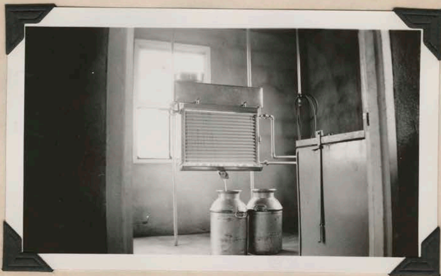
#8 - Milk running over cooler in dairy house #6. Equipped with mechanical refrigeration.
