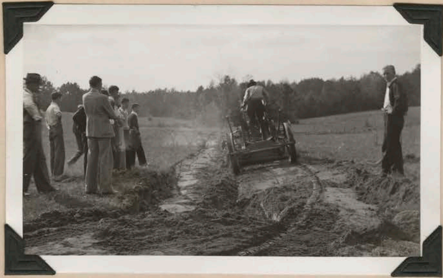
Filling gullies. Halifax county.
