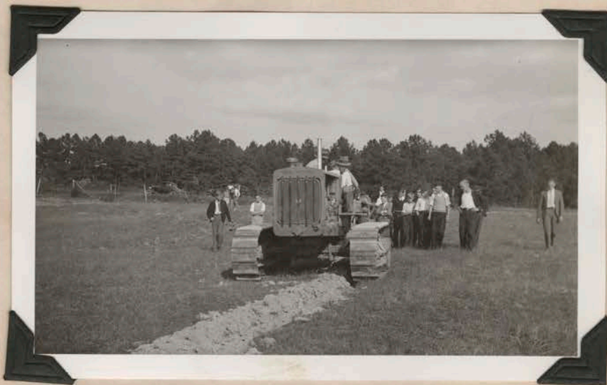
Starting Terrace. Grade line plowed out.
