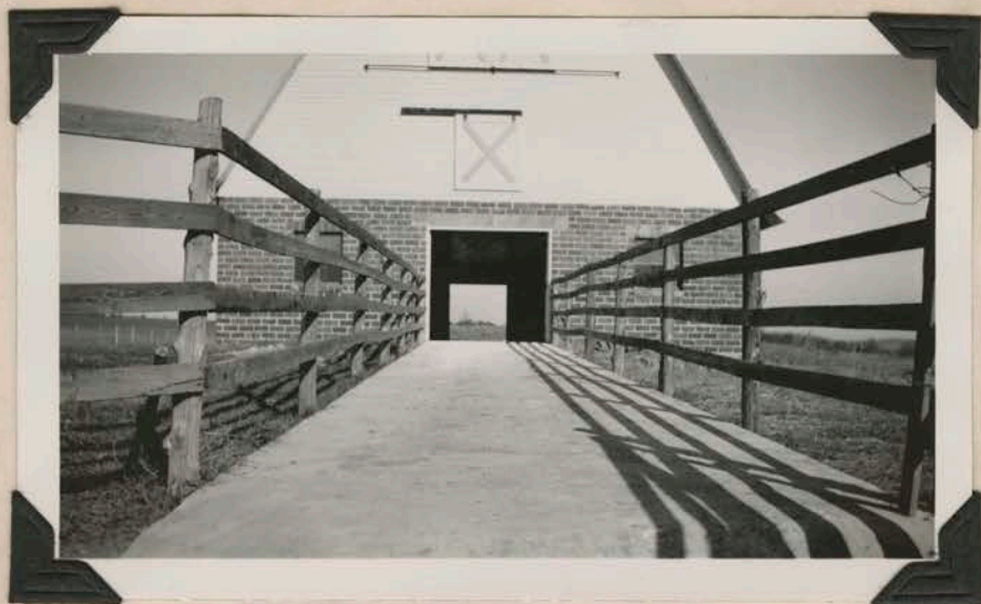
#17 - Fifty foot concrete lane required of Washington shippers.
