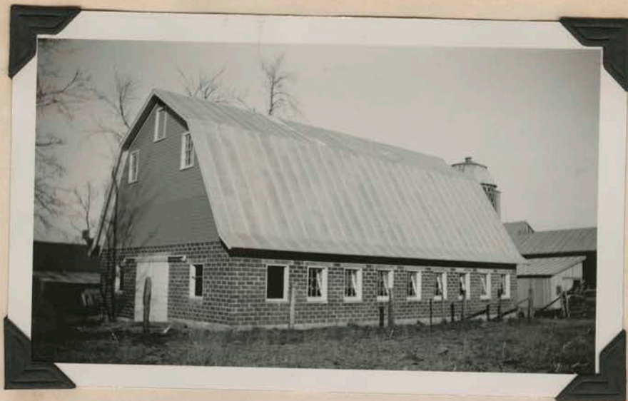
#14 - Tile dairy barn - B-2 - Loudoun county. Under construction.
