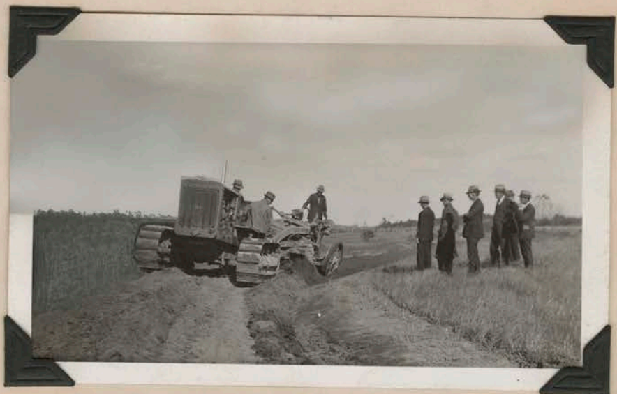
Finishing terrace. Halifax county.
