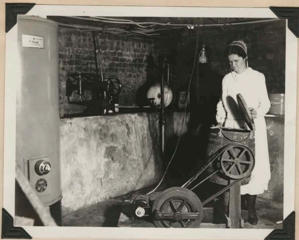
A corner in Mr. S. H. Brunk's basement, showing electric churn, (homemade electric drive) electric water heater, and electric water pump.
