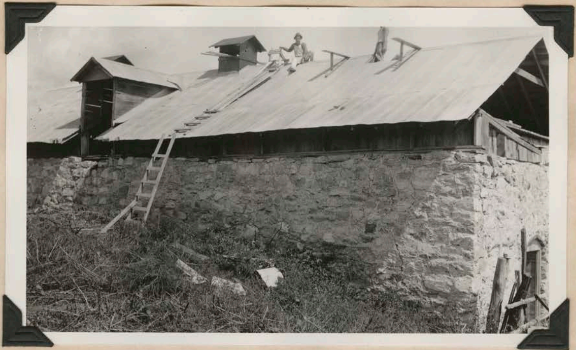
#18 - Old stone silo converted into Irish potato storage of large capacity. Remodeling costs about $600.00.
