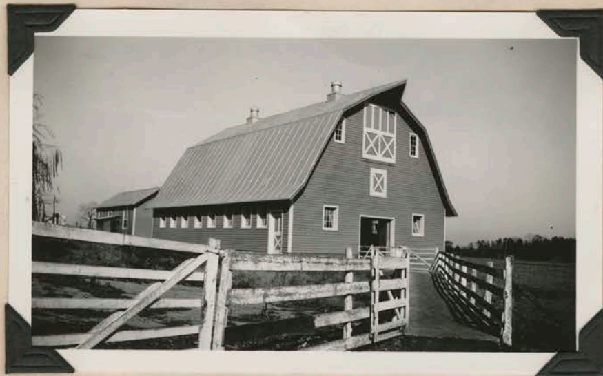
#15 - Frame dairy barn - B-1 - and frame dairy house B-24. Fauquier county. Note 50' concrete lane required by Washington market.
