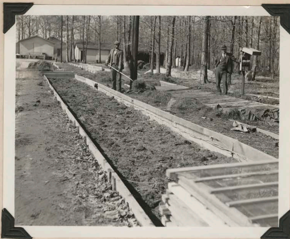
In the foreground, heating cable installed in cold frame to rush spring cabbage. In the background electric hotbeds and meter installation.
