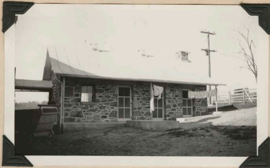
#11 - Stone dairy house with dairy barn #9. Note towels for washing cows' udders hanging out to dry. Washing machines are regular equipment in many dairies supplying Washington market.
