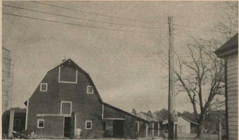
Meter pole and distribution center on a dairy barn in Virginia. There are many advantages and economies in this type of meter installation.
