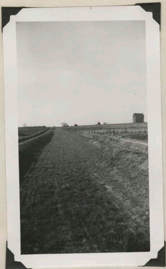
Meadow strip showing side ditches for protection until established
