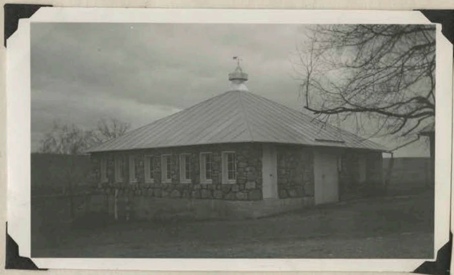
This 16-cow milking barn was built of native stone at a cost of $1,000.00. Rockingham County.
