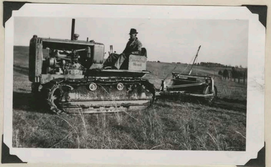
Stream channel cleaning
