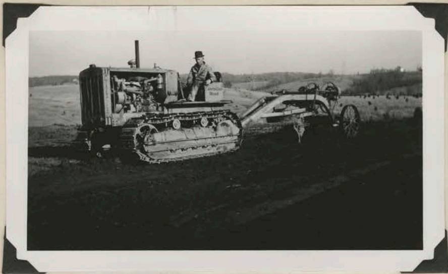
Leveling ridges and ditch
