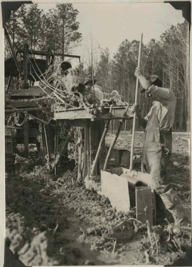
Digging the ditch and laying the tile for drainage in one operation on the Yoder farm.
