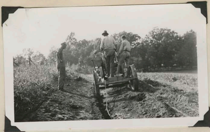
Last cut on terrace channel
