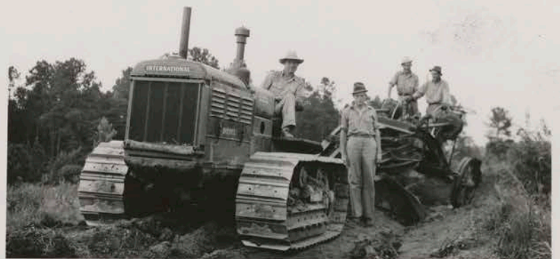
First cuts on terrace
