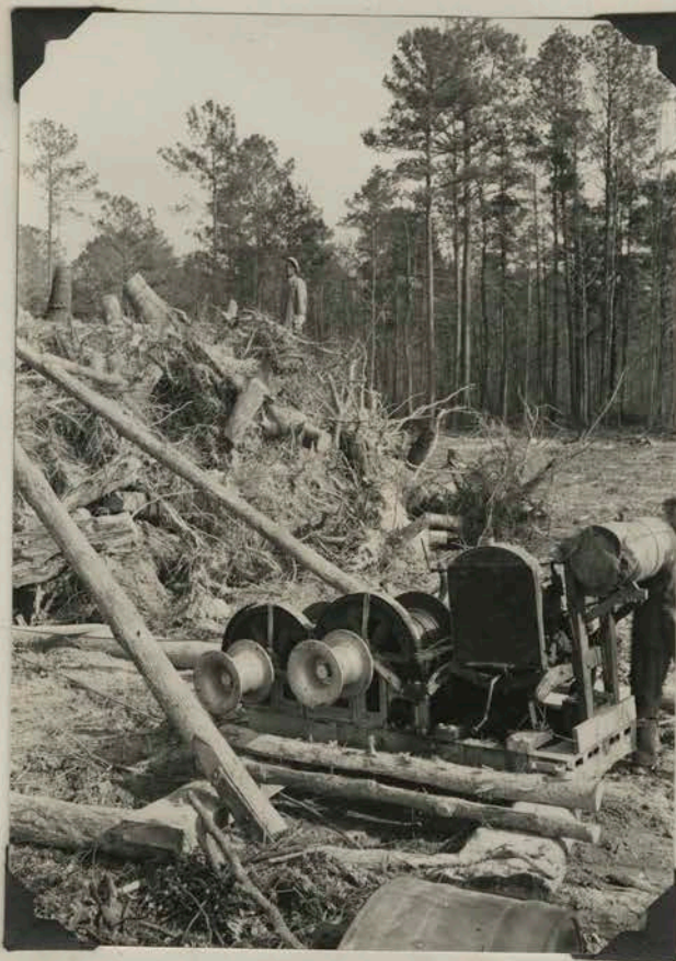
A homemade stump pulling outfit for removing the stumps prior to drainage operations on the Yoder farm, Denbigh, Virginia
