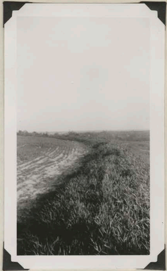
Diversion ditches protecting meadow strip
