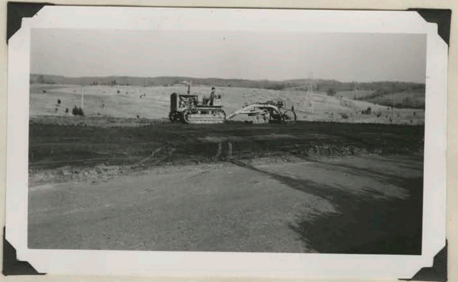
Grading makes up a good part of the demand
