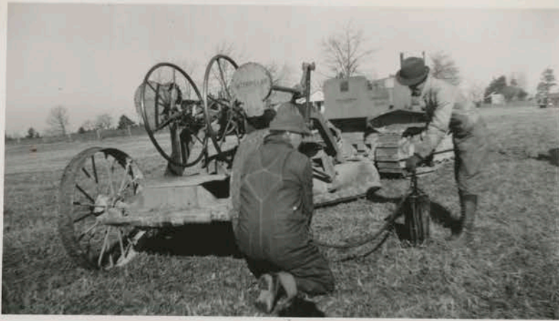
Greasing machinery at start
