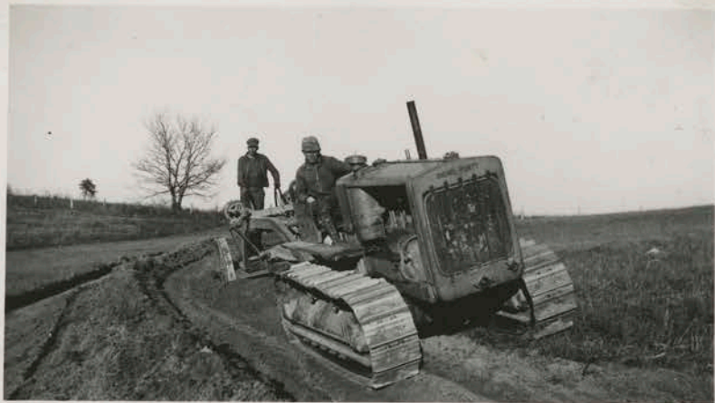
Making back cut on terrace
