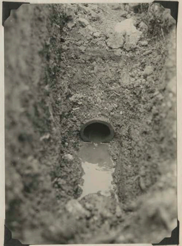
The completed job. Note the flow of the water through tile.
