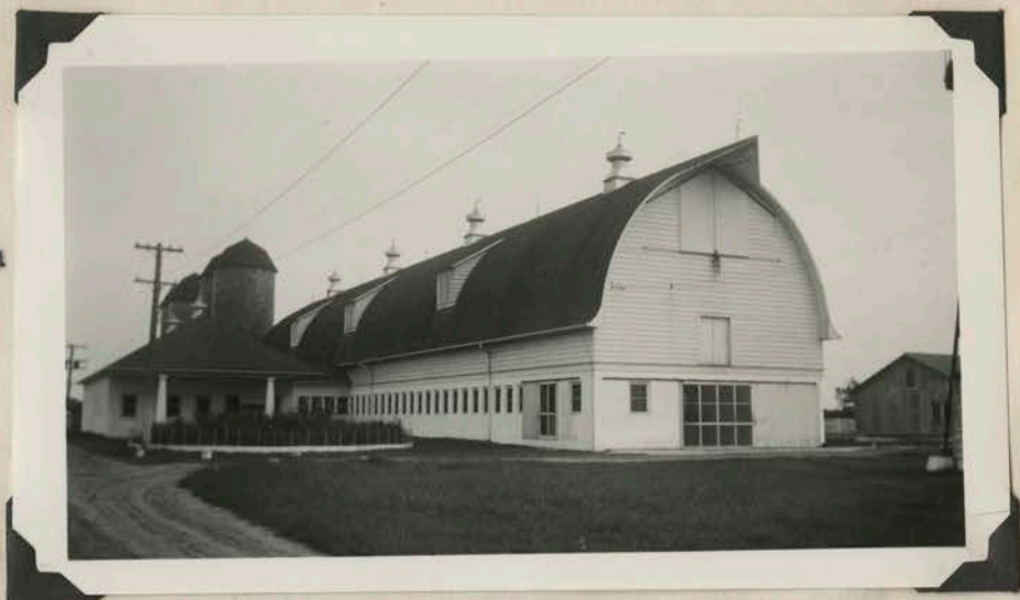
An attractive barn with solid concrete walls, Norfolk area.
