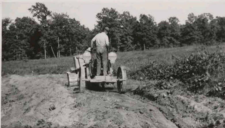
Building terrace channel
