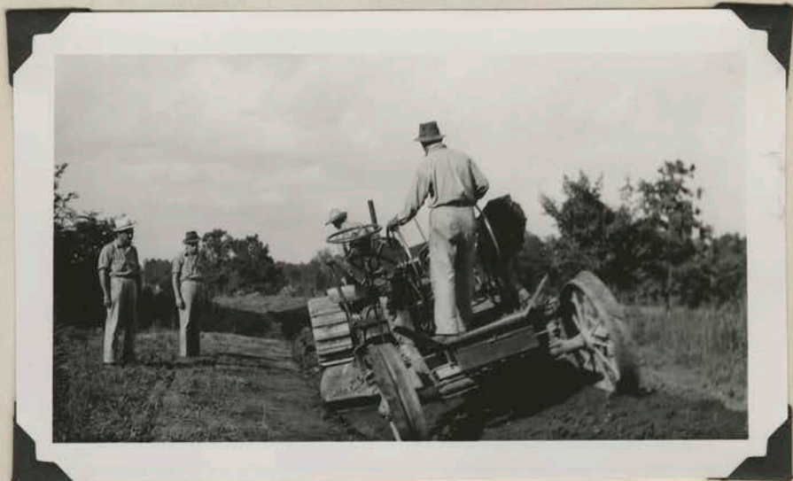
Finishing up terrace channel
