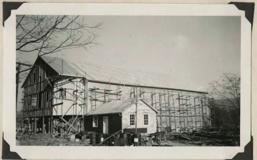
This 30,000 bushel apple cold storage house was built by Graves Bros., Syria, Madison County. Note compressor house in foreground.
