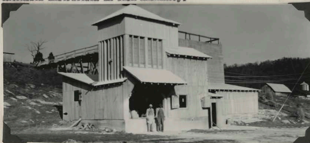
Twin lime kilns. The burnt limestone is run through a crusher, operated with a 20 h.p. electric motor. This plant supplies lime to a large portion of farms in Montgomery County, Virginia.
