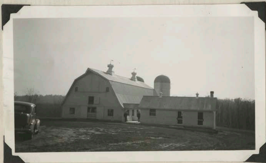
A modern one and one-half story cinder block dairy barn and a three-room milk house painted white. Note relation of milk house and barn.
