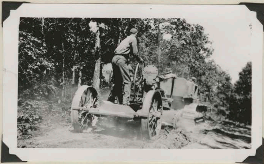
Building farm roads
