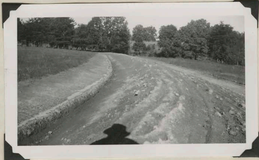
Terrace nearly completed
