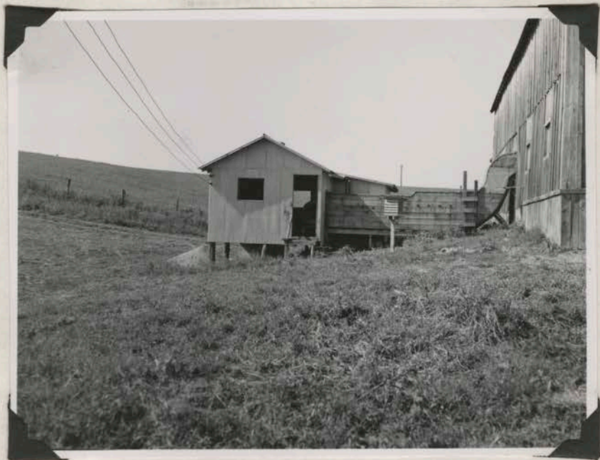
View of building which houses stoker, boiler, fans and controls for delivering heated air into hay mow. The large duct connecting this building to barn contains hot water radiators over which is blown 12,000 cu.ft. of air per minute.
