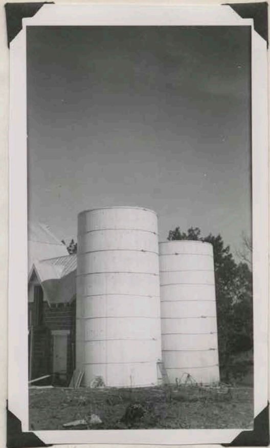
Wood stave silos built of farm lumber cut in local shop. Capacity 22 tons. Approximate cost - $100.00 each.
