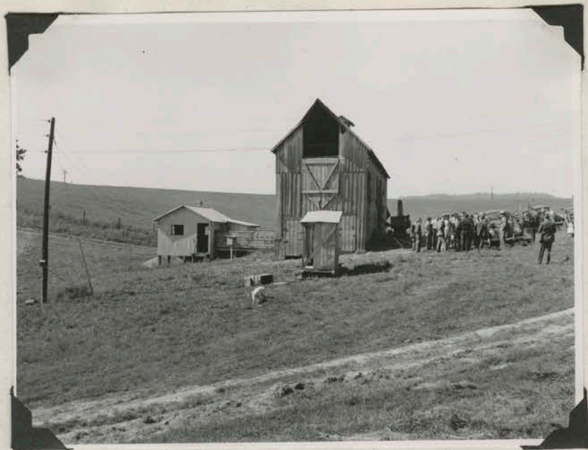
A result demonstration of electric barn type hay dryer in Pulaski County. The small building in the foreground is on skids and houses the hay hoist and 5 h.p. motor.
