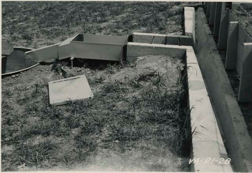
A detail view of concrete catchment trough, approach flume, divisor, and galvanized tank on plots of the new pasture furrow study.
