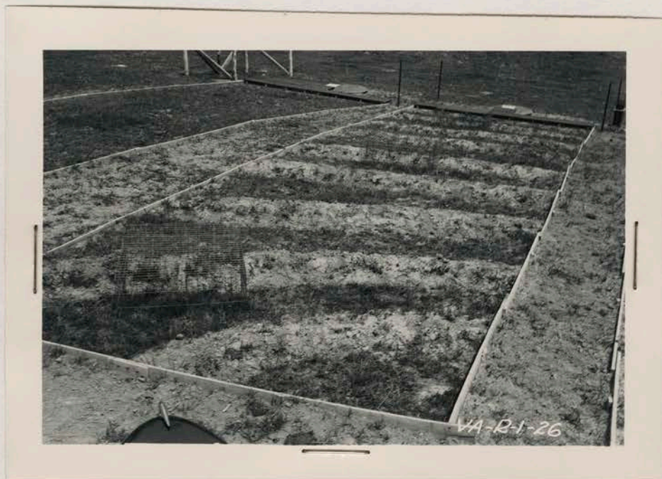
View of newly constructed contour furrows on plot "C" of Block No. 1. Plot "B" is in the background.
