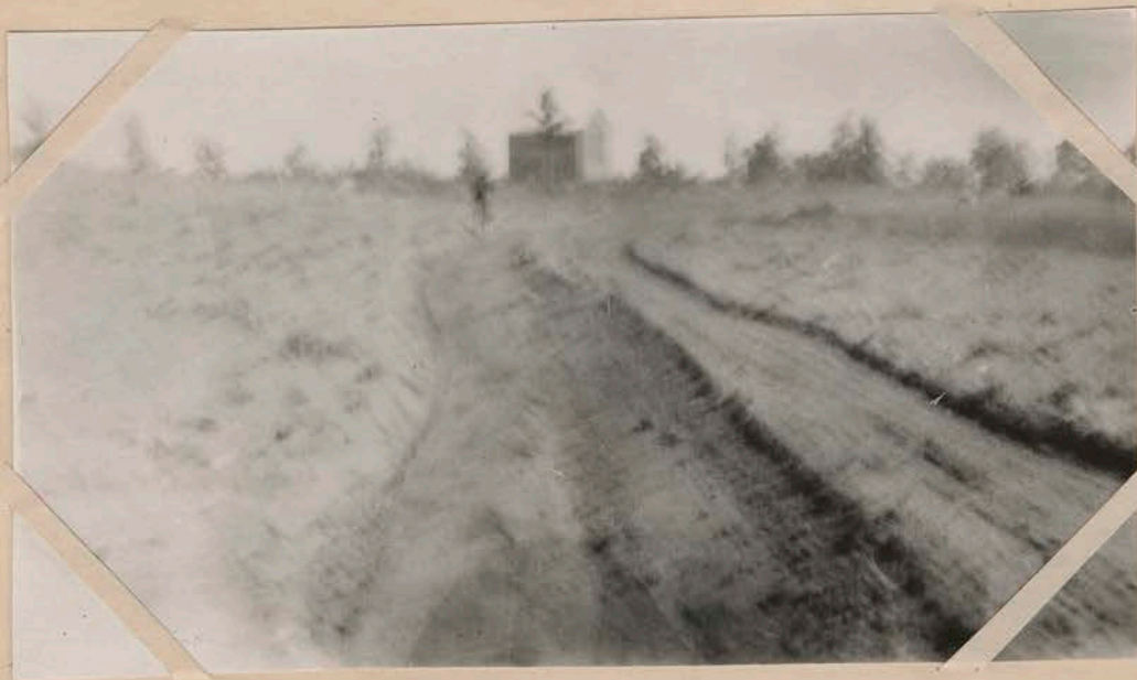
Fig. 5. Terrace in fig. 4. completed. Center of ridge 18 inches higher than base or ground level.
