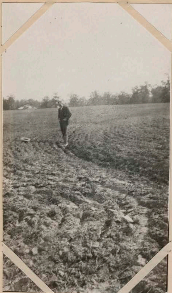
Fig 1 A gullied field two years ago reclaimed by terracing Note terrace
