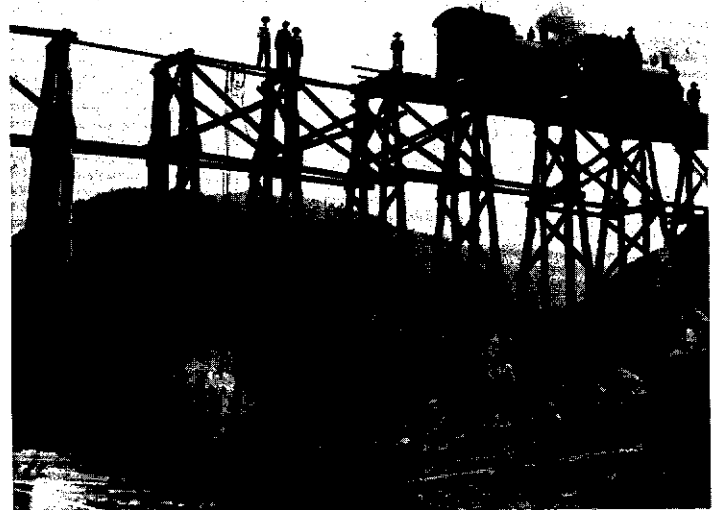
Construction of the Carolina, Clinchfield & Ohio Railroad through Scott County, circa 1907. Pictures courtesy Early Smith (Falls Mills, VA).
