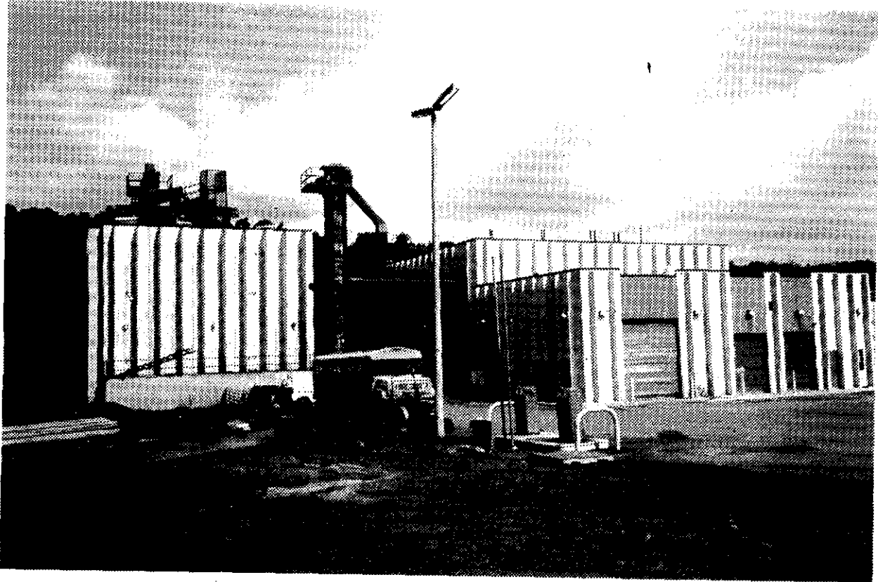
Figure C-1. The Augusta Correctional Center heating plant. The building on the left is for fuel storage. The building on the right houses three wood-waste boilers and attendant equipment.
