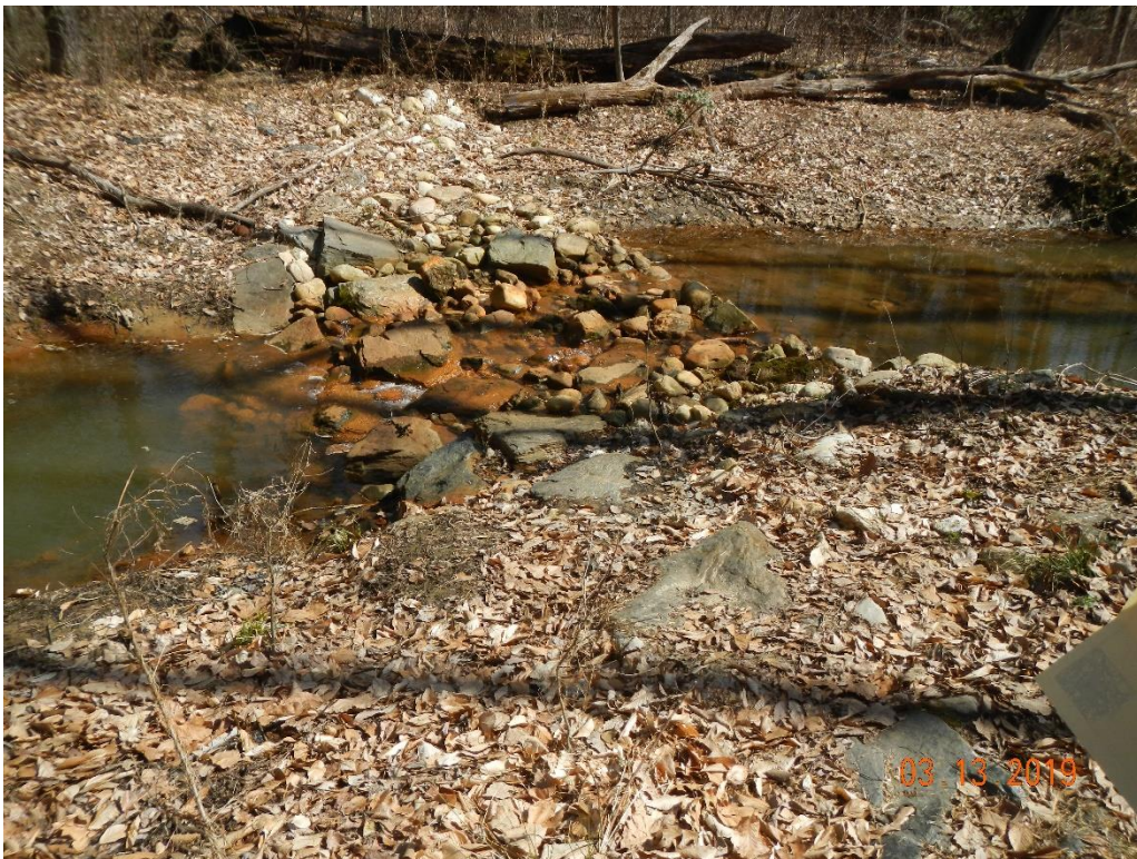
Figure 1. Rock weir implemented in Dividing Creek near Annapolis, MD (taken by Ben Smith).
