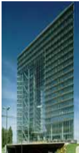
Figure 2.21 South face of “City Gate” (LBNL – http://gaia.lbl.gov/hpbf/picture/ )
