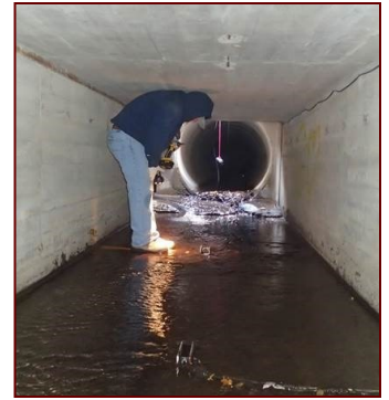
A graduate student inspects a flow sensor in a Blacksburg stormwater pipe.
