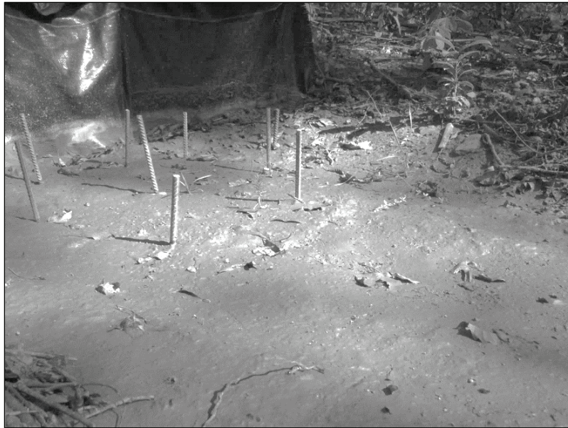
Figure 3. Silt fence catchment area with rebar pins marking the measurement locations.
