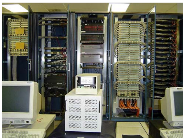
These older racks, with no cable management hardware, also housed modem pool and voice equipment. The new design called for extensive cable management in the racks, as well as consolidating all voice equipment to the ISB switchroom.
