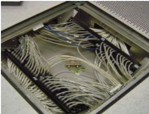
Old Floor Box
