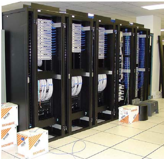
The new equipment is fully cabled and service is in transition.
