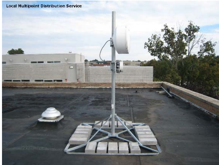
Town Centre LMDS Roof Antenna Mount with Ceragon one-foot dish
