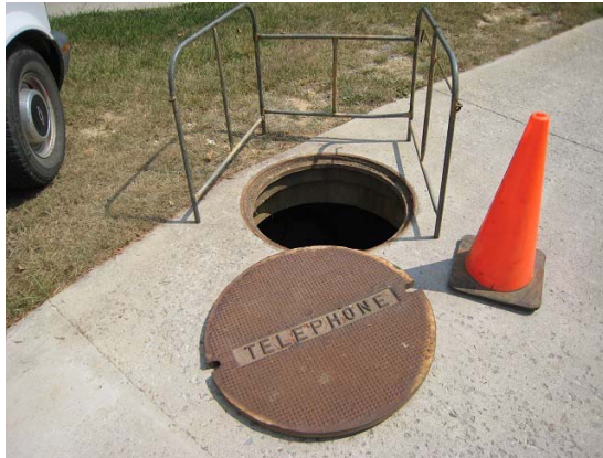
Maintenance hole for pulling underground cables and splicing them together
