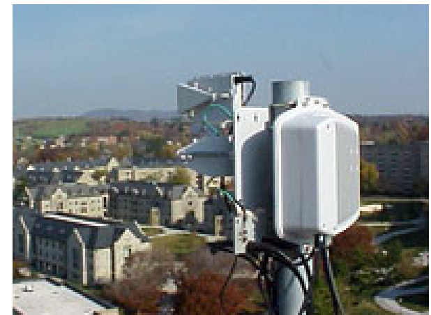
Harris-WavTrace LMDS multipoint nub deployed at Virginia Tech
