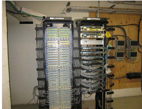
Main telephone equipment room in a newer building
