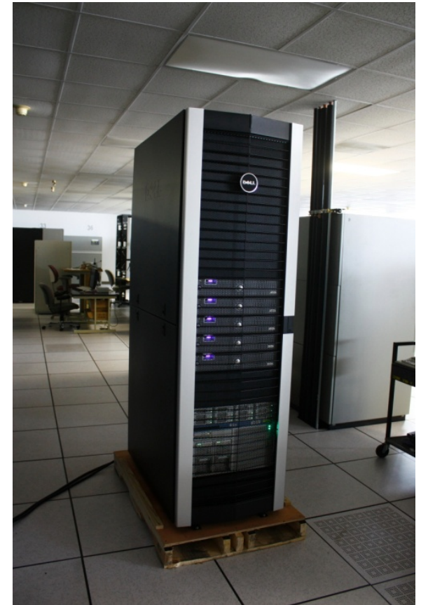
Disaster recovery equipment
