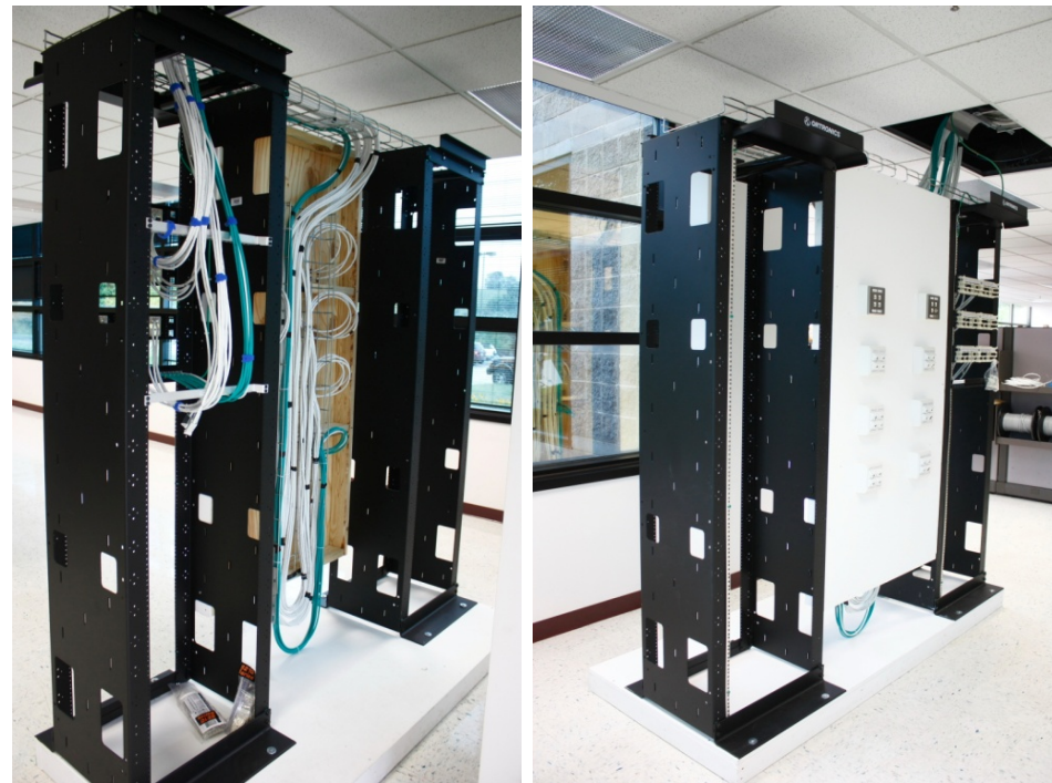
Cat 6A test bed
