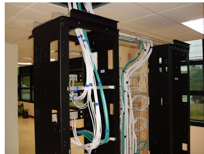
Test setup for new cables and connectors that support 10 Gbps to workspaces
