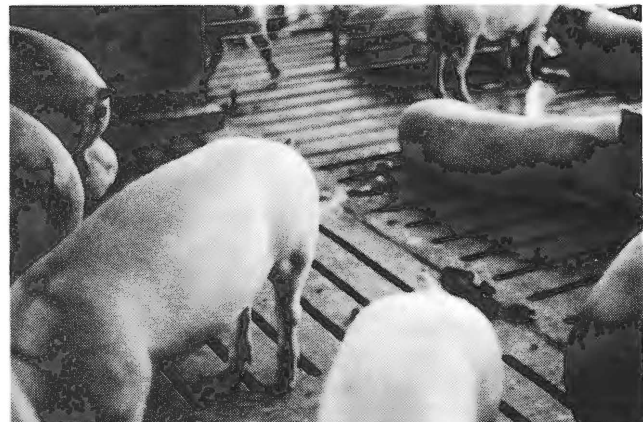
Figure 4. Slotted floor in swine confinement building.
