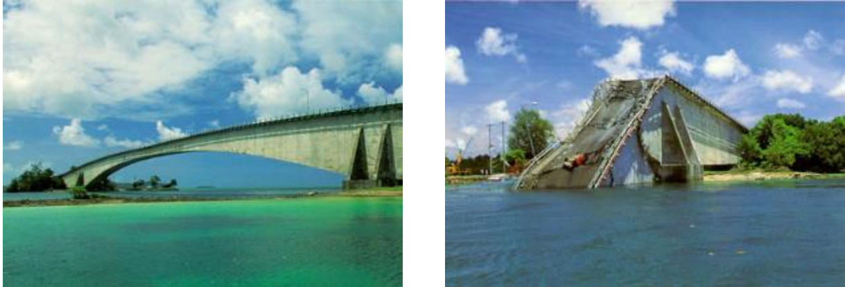
Figure 1.1. (Left) Koror-Babeldaob Bridge prior to collapse. (right) Koror-Babeldaob Bridge after collapse. (OPAC 2000)
