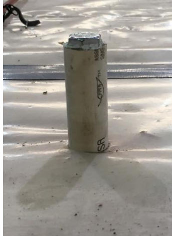
Figure 19. Whiffle Tree Blockout
