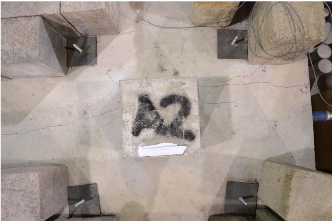
Figure H.46. Column A2 after Testing
