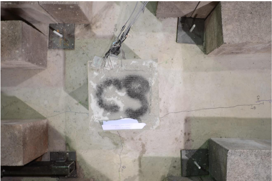
Figure H.48. Column C3 after Testing
