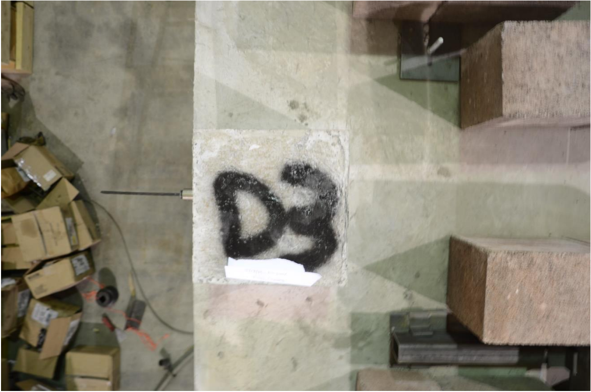
Figure H.47. Column D3 after Testing
