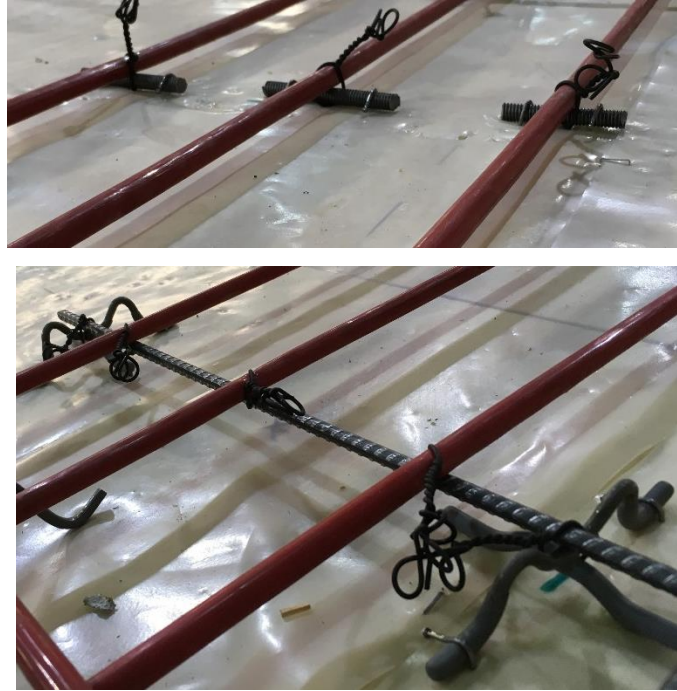
Figure 20. Banded Tendon Slab Chair Examples
