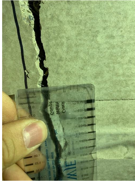
Figure 74. Crack Width Measurement at Bottom Crack
