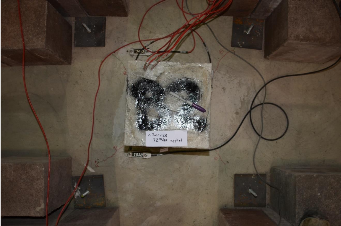
Figure H.23. Column B2 at Service-Level Loading
