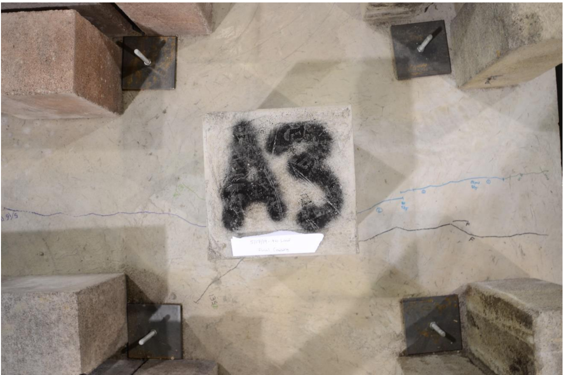
Figure H.50. Column A3 after Testing
