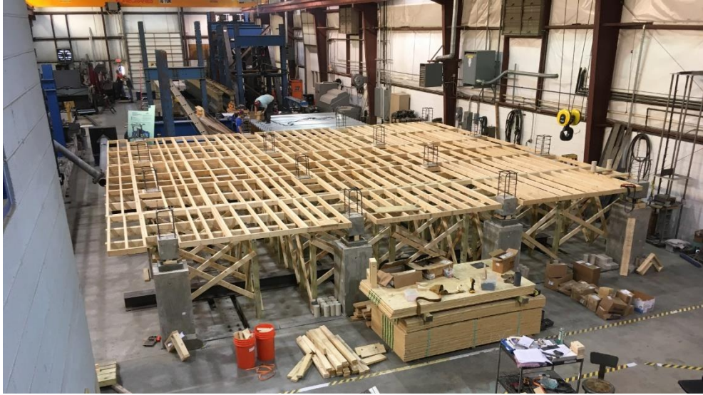
Figure 18. Scaffolding at Early Stage
