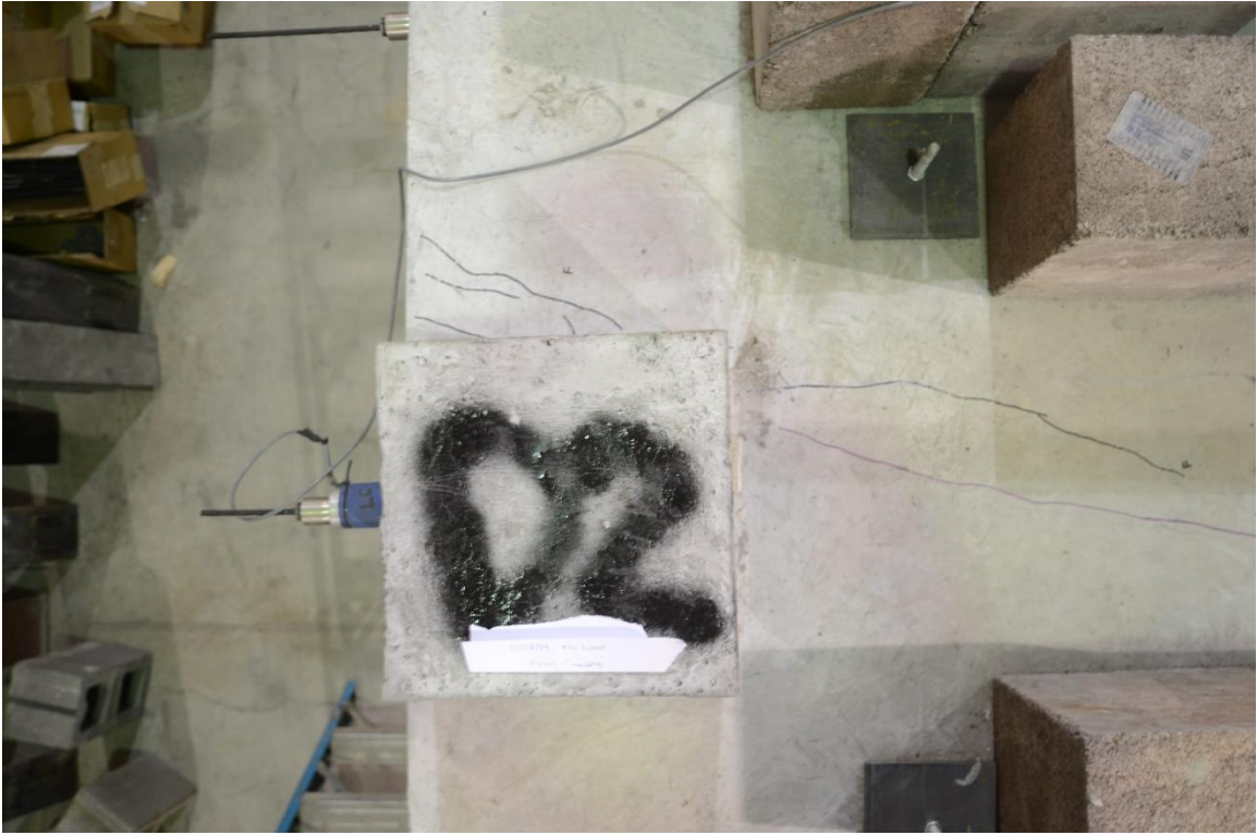
Figure H.43. Column D2 after Testing
