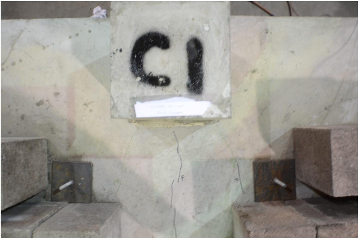
Figure H.40. Column C1 after Testing
