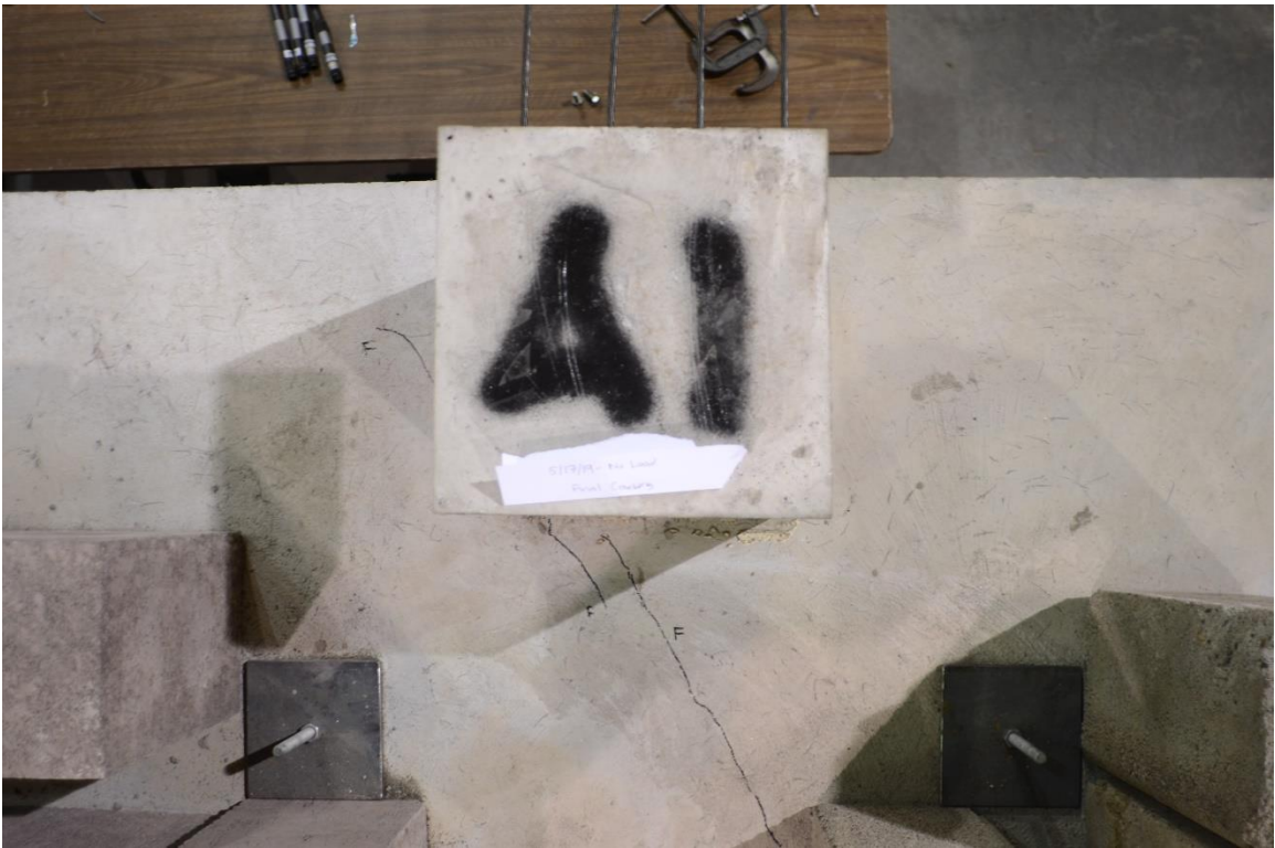
Figure H.42. Column A1 after Testing
