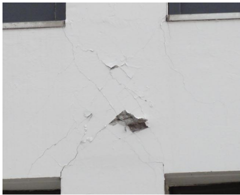
(a) Shear crack observed in 2011 Christchurch earthquakes (Leon et al. 2014);
