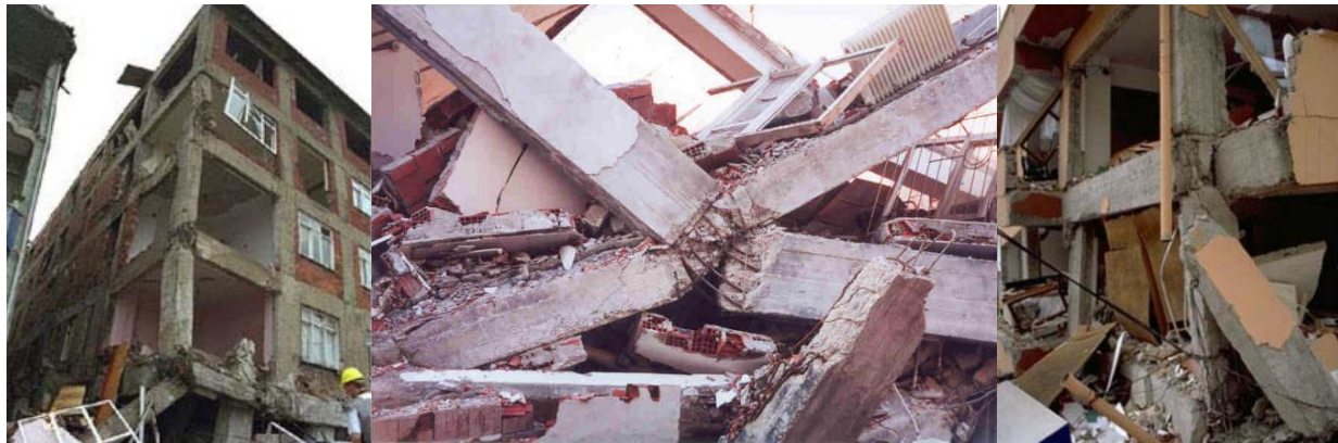
Figure 1-1 Damaged BCJs in non-ductile RC frames (H. Sezen et al. 2000)
