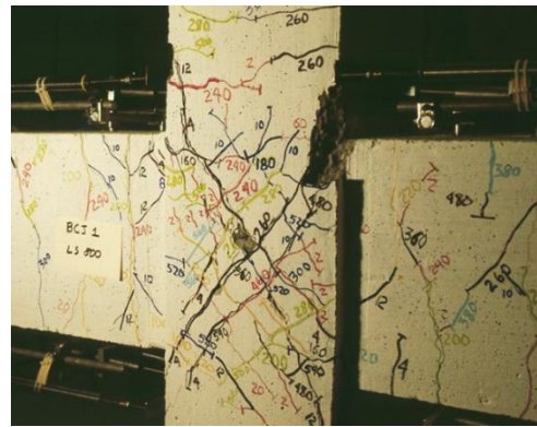
(b) shear crack observed
