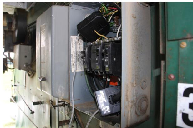
**Fig 15. Two current transducers measured total current and motor current respectively**
