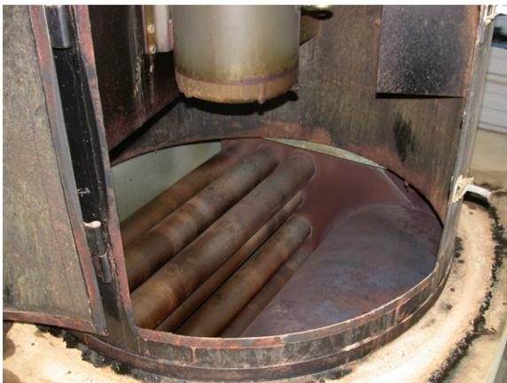
**Fig 4.** Heat exchanger assembly of a gas furnace.
