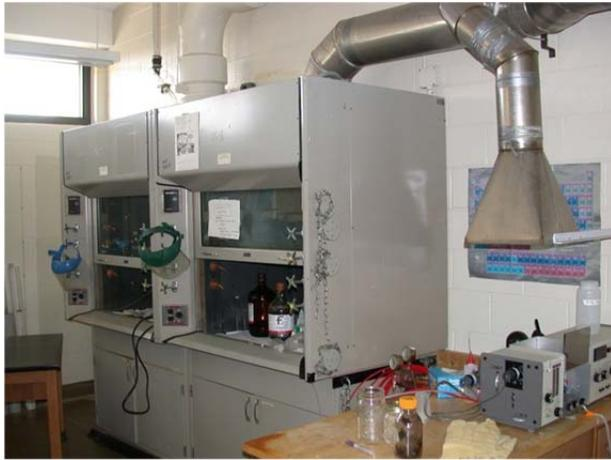
Fig. 2 Original configuration of fume hoods with vertical sash mechanism in DER 5065.
