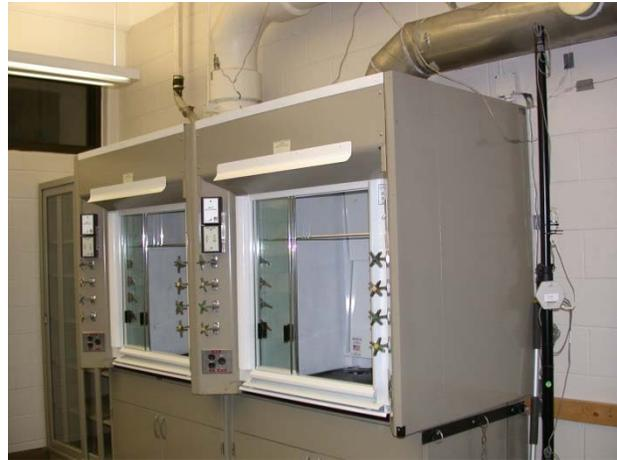
Fig. 3 Retrofitted fume hoods with new VFV control system, safety cabinet, and vertical sashes.
