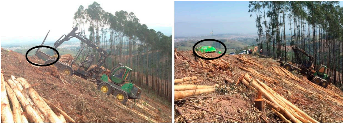
Figure 2. HAAS machine-mounted traction winch, circled left, and T-WINCH self-contained traction winch, circled right, used in conjunction with a John Deere 1910E forwarder.
