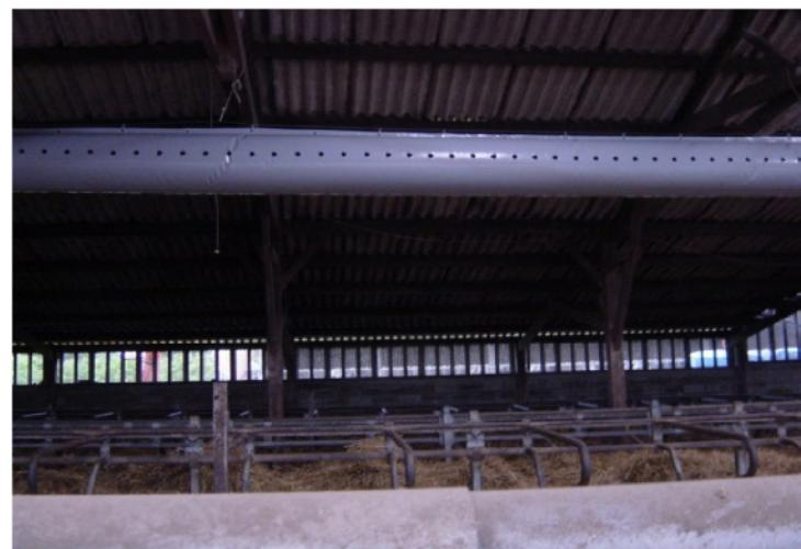
**Figure 7.** Duct for dispersing an artificial tracer gas within an animal house.
