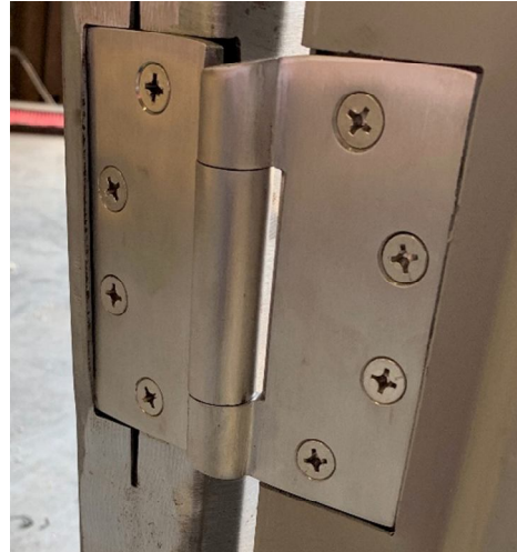
(b) Series 9A typical hinge attached to deformed hinge reinforcement plates.
