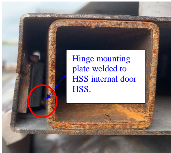
(a) Beam-assembly hinge mounting plate.
