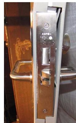
(c) Typical latch strike plate failure via dynamic testing.
