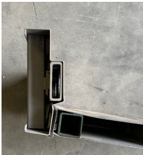
(a) Series 9B weld failure and frame-skin deformation.
