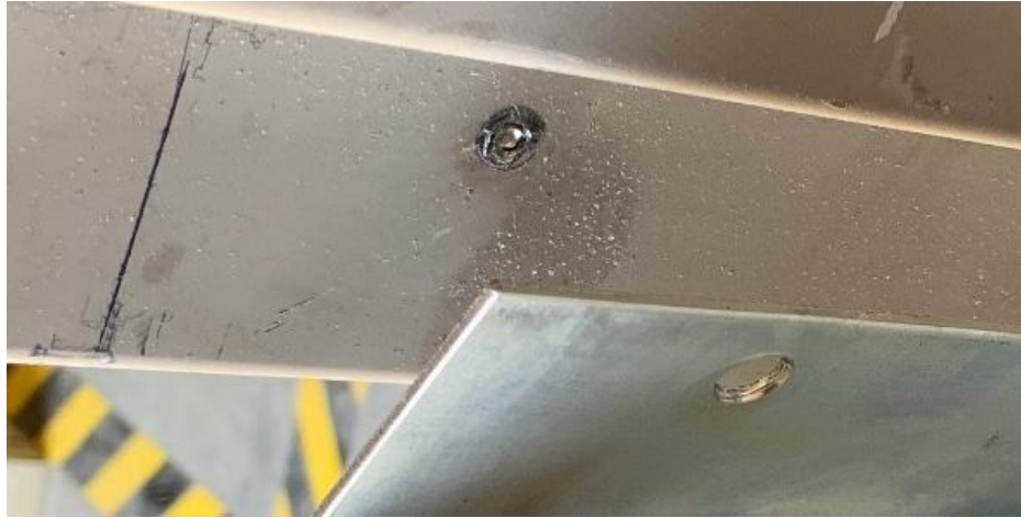
(a) Typical Series 7 screw shear failure (on frame side).
