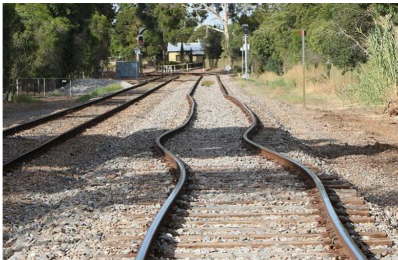
Figure 2.3: Buckling of tracks in lateral direction [9]
