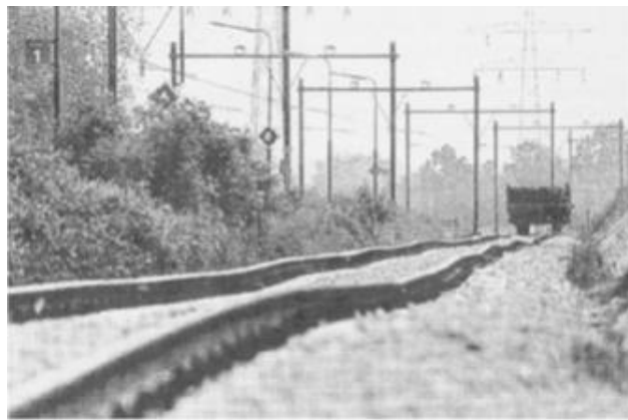
Figure 2.2: Defects in railway track geometry [8]
