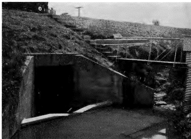
This runoff gaging station located on Powell's Creek in Halifax County, uses a Virginia V-notch weir for low-flow measurement and, in the corrugated stilling well at the right, an automatic flow depth recorder. A 1.3" per hour runoff from the 182-acre watershed has been recorded.
