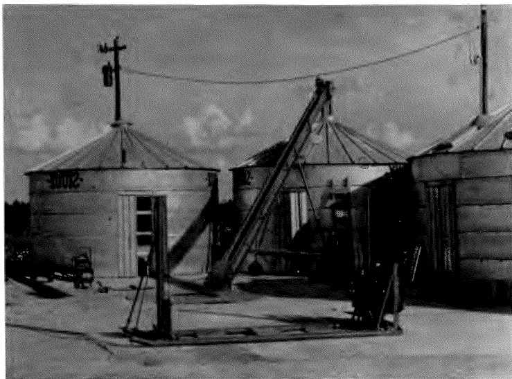
A typical farm installation for artificially drying and mechanically handling windrow-harvested peanuts.
