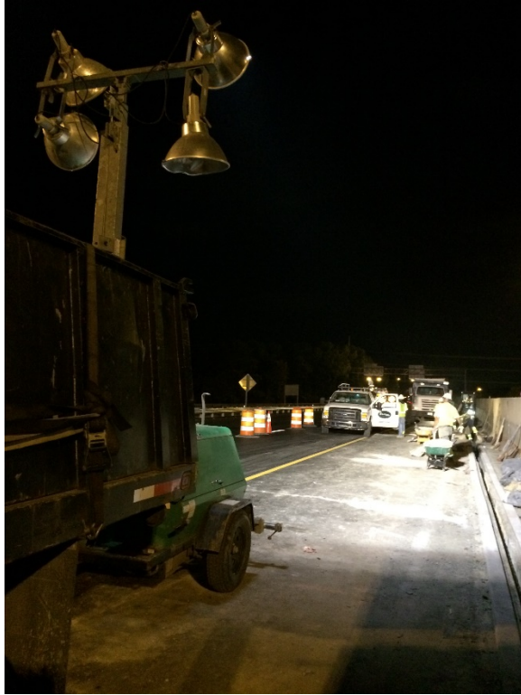
Figure 18. Metal halide light tower at the trench drain installation on I-64 west.
