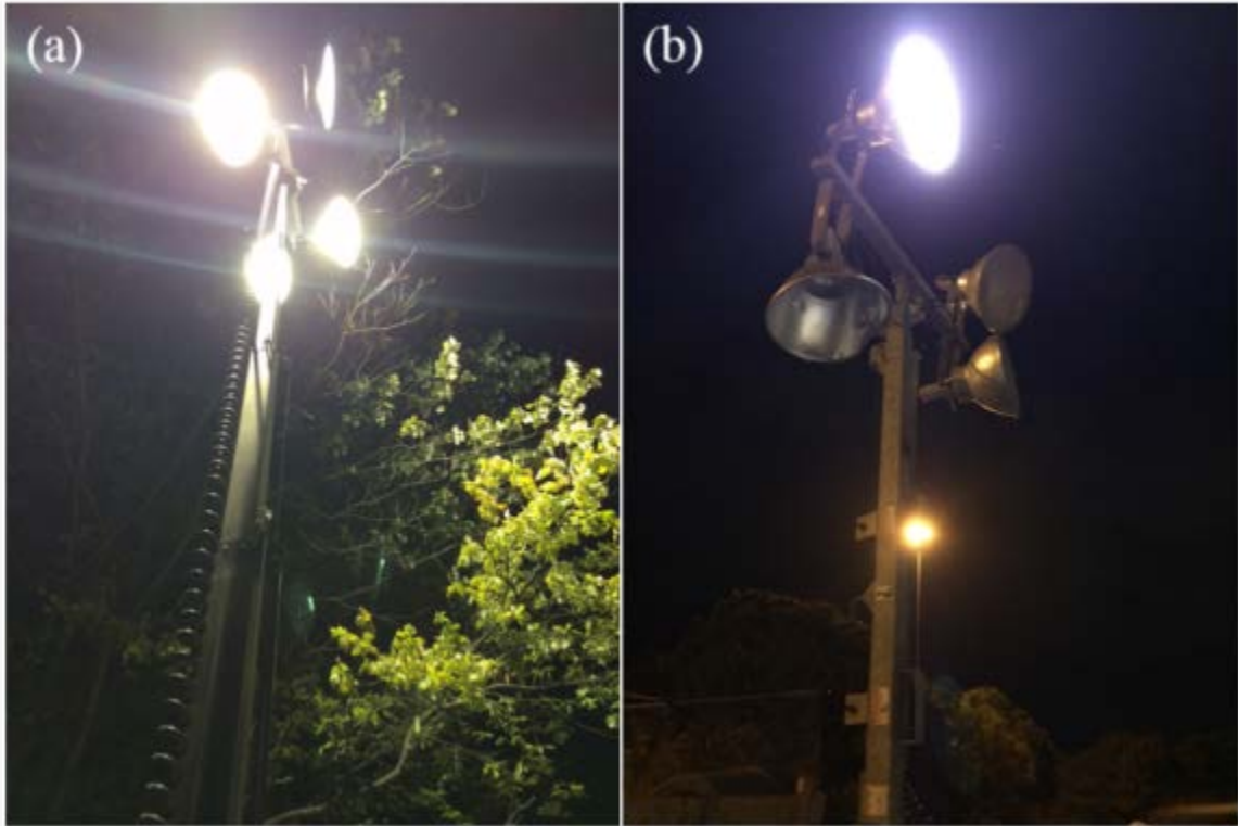
Figure 26. Metal halide portable light towers. (a) All four luminaires powered on at bridge work (I-81 N). (b) One luminaire powered on at a trench drain installation (I-64 W).
