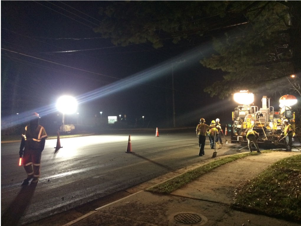
Figure 24. Balloon light towers on the paver (right) used in conjunction with the metal halide portable light tower (left) on VA-674.
