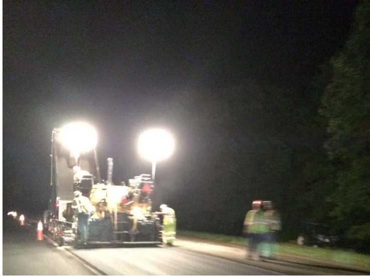
Figure 12. Balloon light towers at the I-81 north milling and paving work zone.
