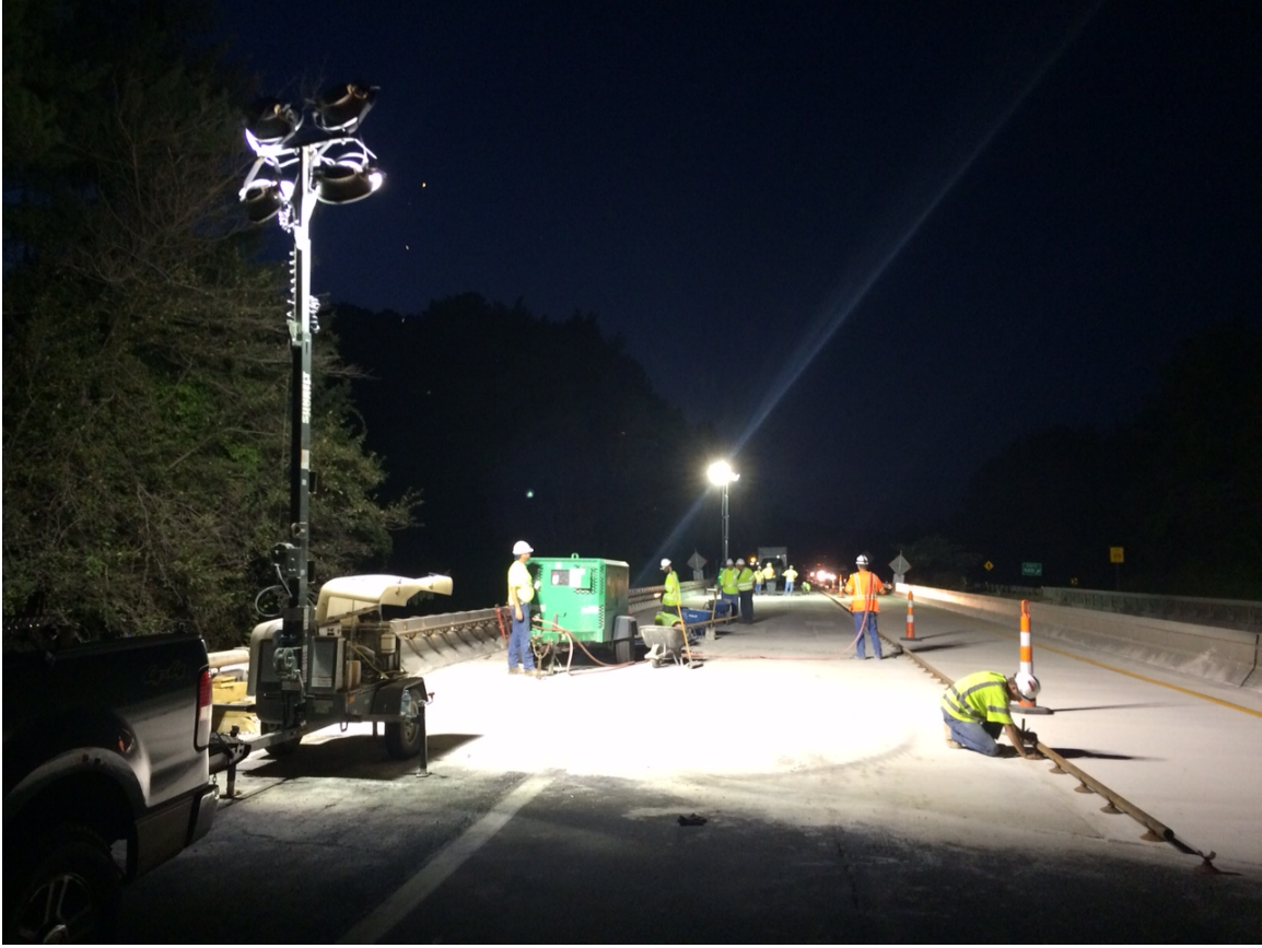
Figure 8. Metal halide portable light towers on I-81 south bridge work.
