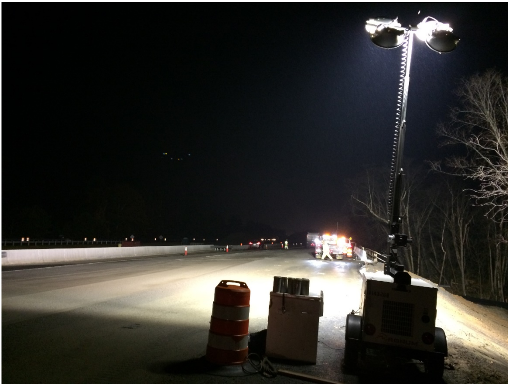
Figure 20. Metal halide light tower at the road widening operation on I-64 east.
