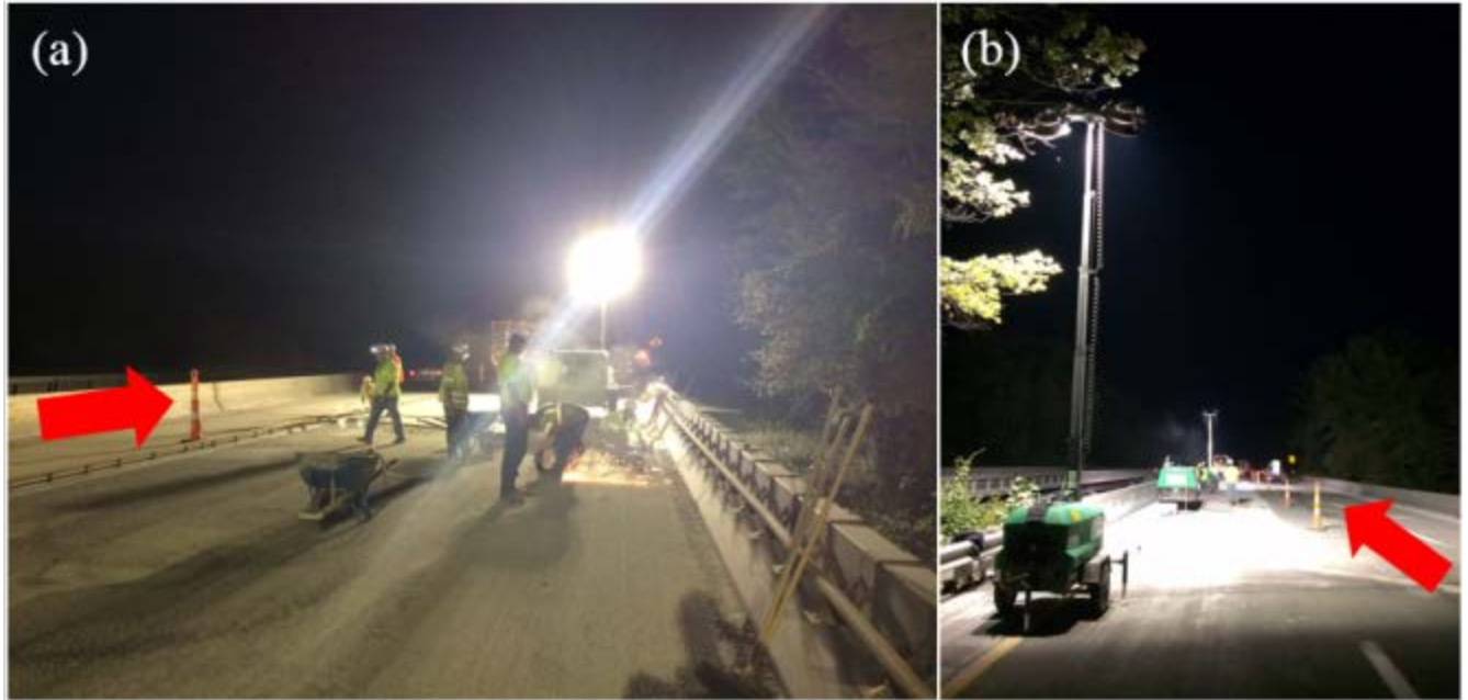
Figure 32. Aiming of the luminaires on portable light towers and resulting significant changes in the vertical illuminance levels in the work zone. Red arrows= direction of traffic flow. (a) Light tower aimed toward traffic, resulting in higher mean and maximum vertical illuminance levels ( M = 22.68 lux and Max = 122.2 lux). (b) Luminaires aimed away from the traffic, resulting in lower mean and maximum illuminance levels ( M = 0.88 lux, Max = 14.91 lux).
