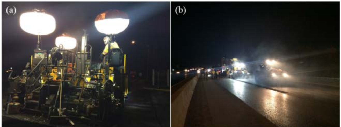
Figure 27. (a) Balloon light towers. (b) LEDs mounted on pavers and rollers.
