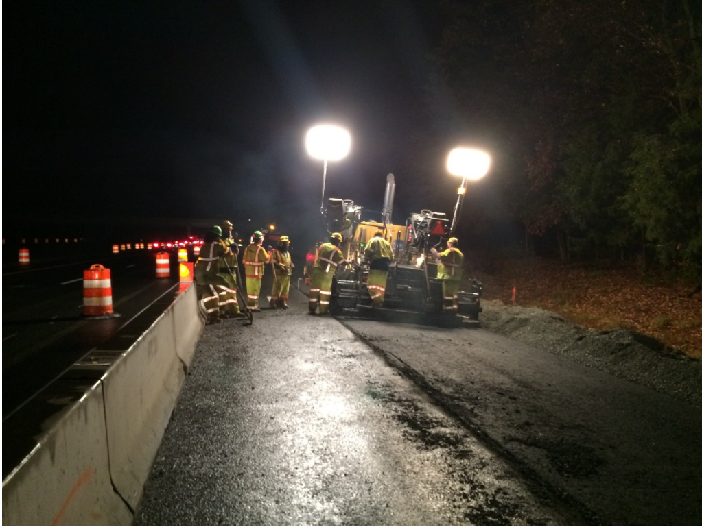
Figure 22. Balloon light towers at the paving operation on I-64 west.
