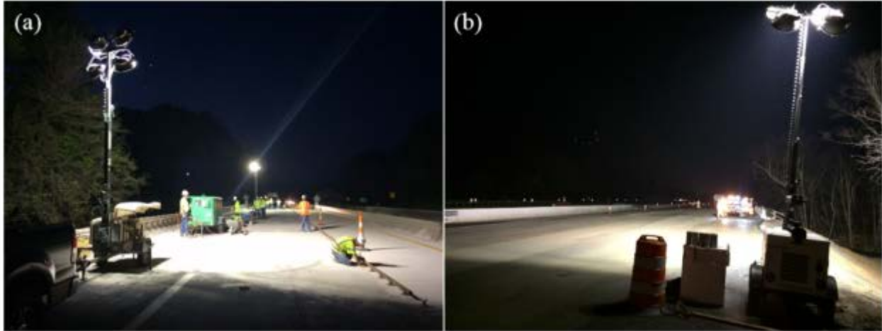
Figure 29. Horizontal illuminance level in the travel lane as a result of location of portable light tower and number of light towers. (a) Higher horizontal illuminance levels in travel lane than in (b) with fewer light towers and more lanes.
