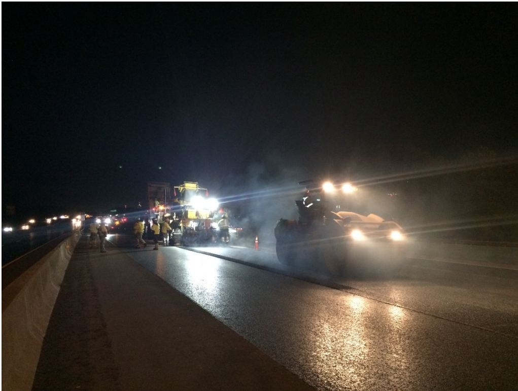
Figure 16. Vehicle mounted LED lights being used to illuminate the work area in the milling and paving operation on I-264 west.
