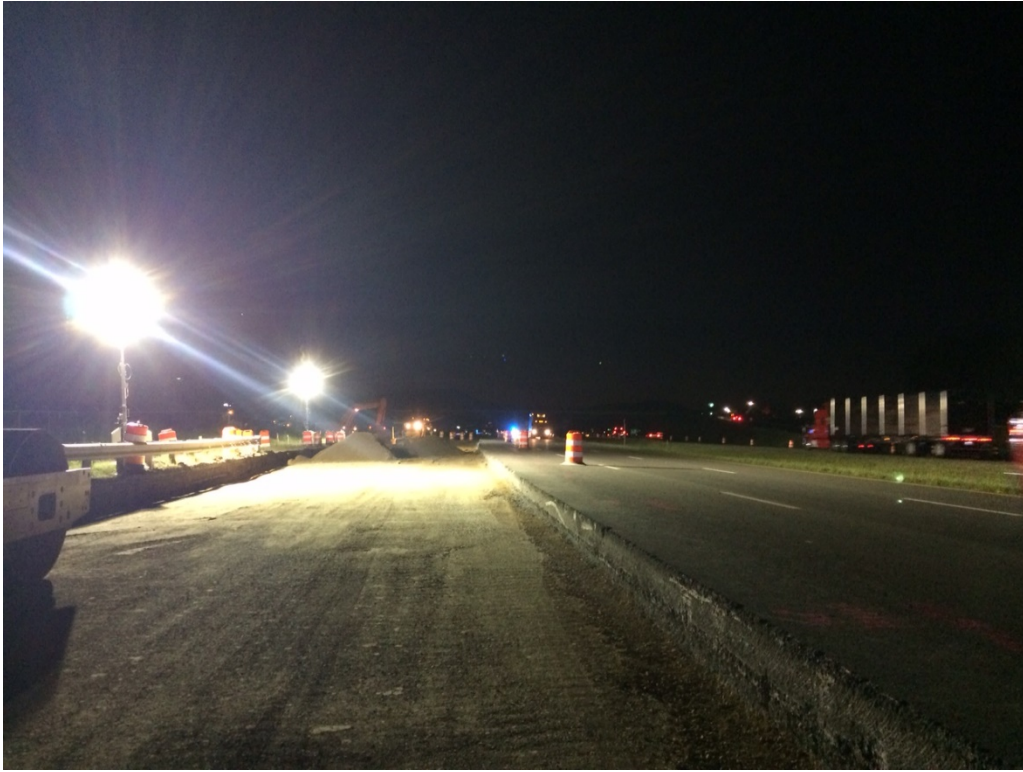
Figure 14. Metal halide portable light towers at the I-581 south on-ramp work.
