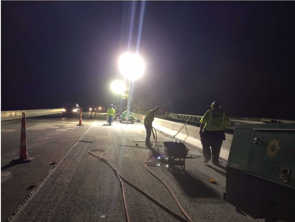
Figure 10. Metal halide light towers aimed away from the traffic at the I-81 north bridge work.
