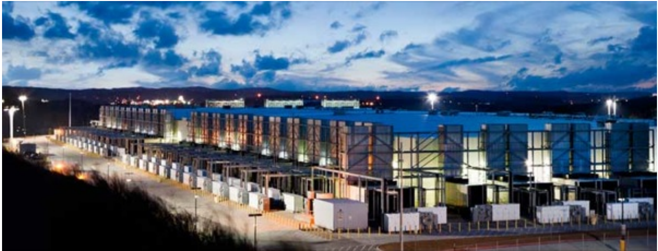
Figure 1.2: A modern data center.
