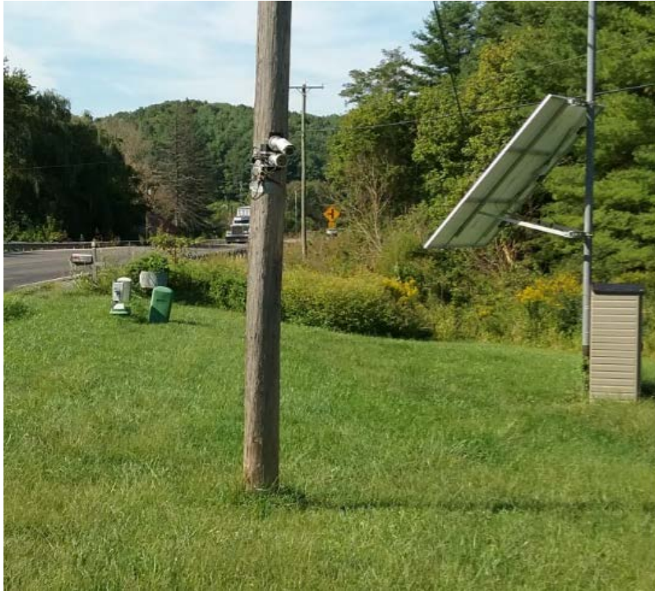
Figure 12. Surveillance Camera ( Top ) and Illuminator Used for Cable/Site Monitoring. The Solar Power System ( Far Right ) and Processor Enclosure ( in the Background ) are also Shown.
