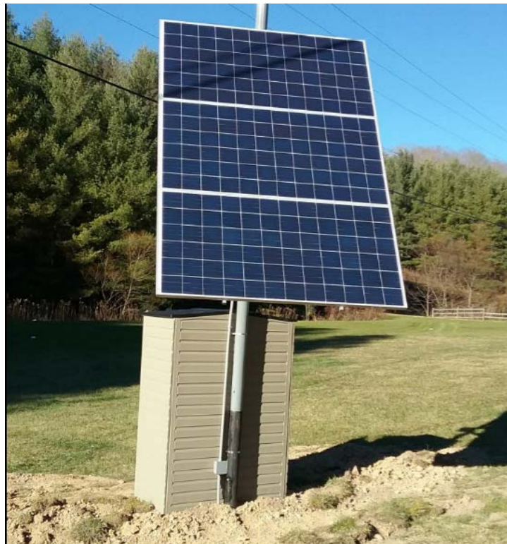
Figure 9. Solar Photo-voltaic System Supplying Power to the Buried Cable and Surveillance Equipment.
