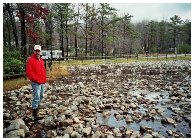
Fig. 8 Limestone leach beds add alkalinity to fresh water, which can then be mixed with AMD for treatment (Photo: J. Skousen)
