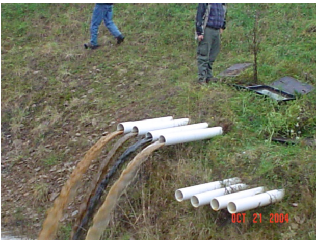
Fig. 5 Flushing systems can be placed at the outlet of VFWs to remove accumulated flocs in limestone. (Left) an operator opens a below-ground flushing valve; (right) flushed water emerges with visible flocs (Photos: J. Skousen)
