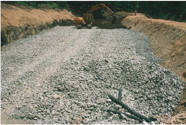
Fig. 4 Vertical flow wetlands have perforated pipes embedded in a limestone layer at the bottom of the system and overlain by organic-matter substrate. Water is ponded on the surface which drives the water through the substrate, limestone and out through the pipes. (Photos: J. Skousen)
