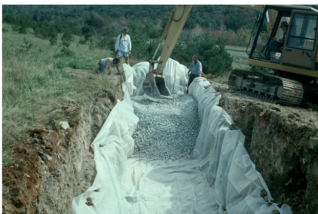
Fig. 6 Anoxic limestone drains are buried trenches of limestone. Care must be taken to introduce anoxic water with low Al concentrations (Photo: J. Skousen)
