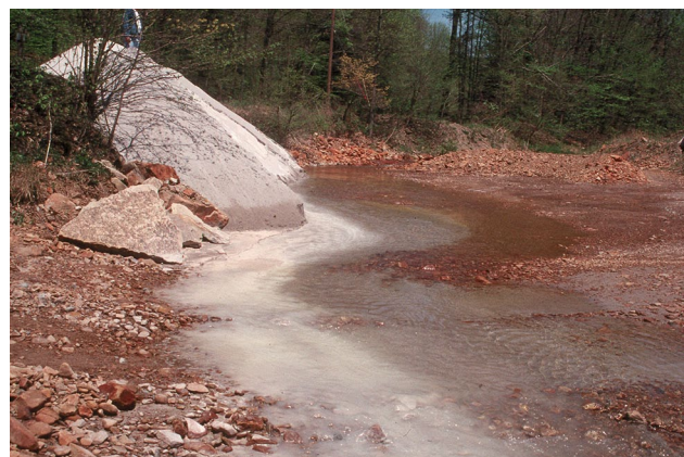
Fig. 10 Limestone sand can be placed in polluted streams to treat AMD. The turbulence in the stream aids limestone dissolution and minimizes metal-precipitate armoring, improving its effectiveness (Photo: J. Skousen)
