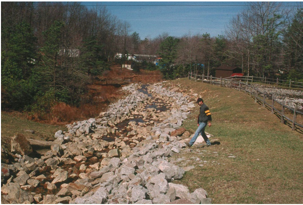
Fig. 7 Open limestone channels are streams or ditches lined with limestone rock. Although the limestone becomes coated with precipitates, dissolution and acid neutralization continues but at lower rates than for uncoated limestone rock (Photo: J. Skousen)
