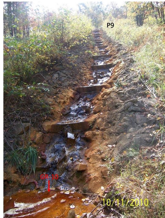
Fig. 11 Low pH Fe oxidation channels can remove Fe concentrations in water even when water pH is low (Photo: T. Danehy)
