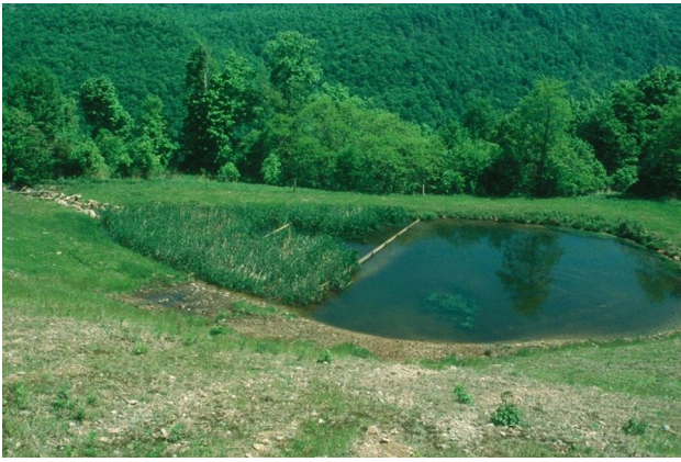
Fig. 2 Aerobic wetlands are best suited for net-alkaline water where Fe and Mn are oxidized, precipitated and captured. The metal hydroxides are collected and retained in wetland substrates. (Photo: J. Skousen)
