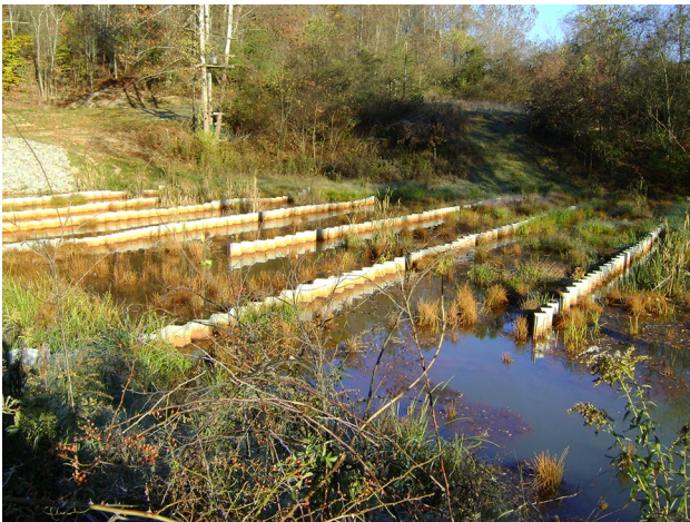
Fig. 3 Anaerobic wetlands can treat net-acidic water because microbial sulfate reduction and limestone dissolution generate alkalinity (Photos: J. Skousen)
