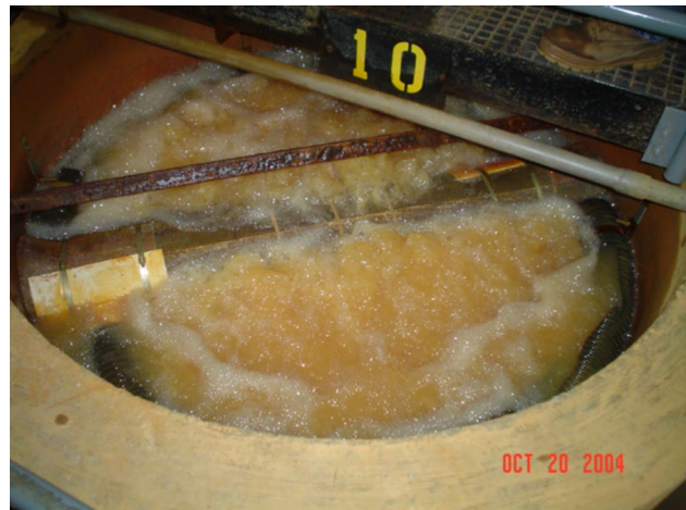
Fig. 9 Diversion wells are cylindrical concrete or metal tanks filled with limestone. A metal pipe extends down the length of the tank and carries AMD to the bottom of the tank under pressure to agitate and fluidize the limestone in the tank to minimize coating and enhance dissolution (Photo: J. Skousen)
