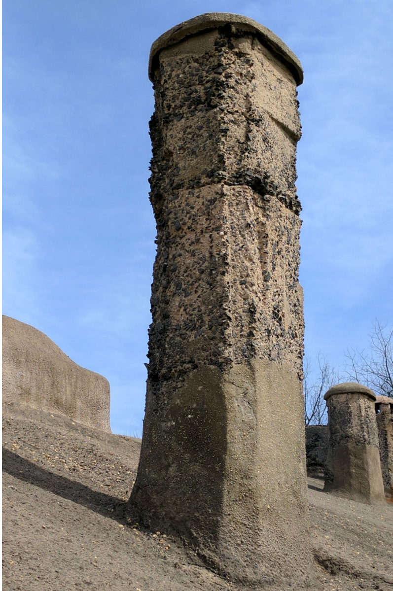
Figure 1.19. Chimney at the Moravian Pottery, with cement render waterproofing. Image: author.
