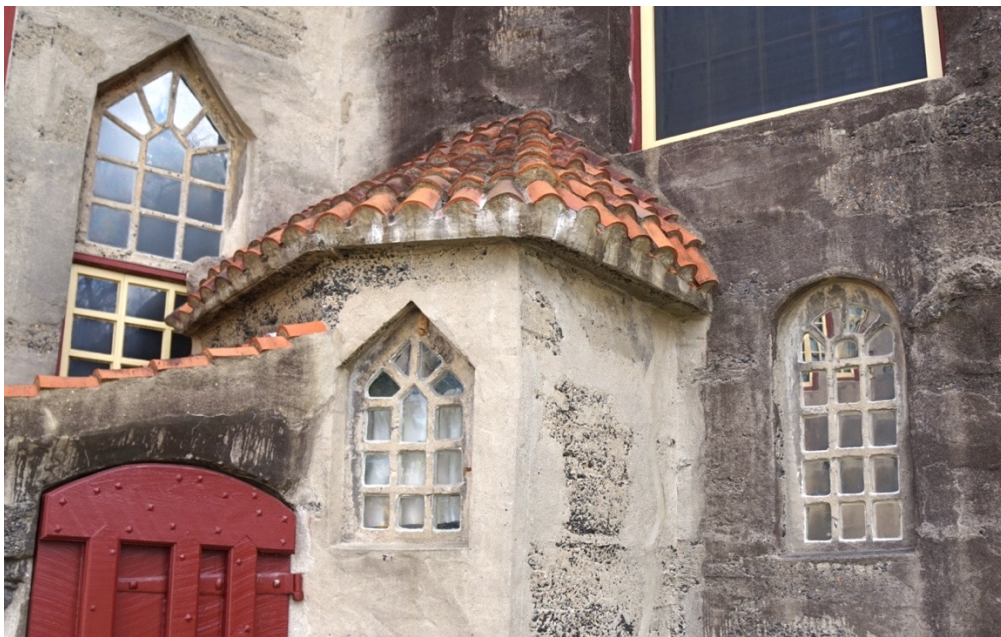
Figure 3.18. Rear facade of Fonthill, present day. Image: author.
