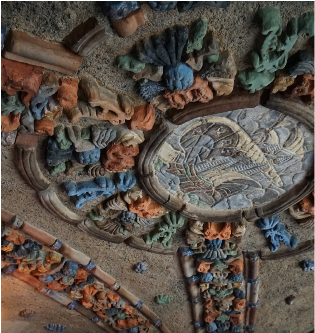
Figure 6.10. Typical sand-form finish, with embedded tiles, at the Fonthill library ceiling. Image: author, courtesy of Fonthill Castle.
