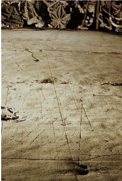
Figure 2.27. Tracing Room Floor at York Cathedral. Note the templates in the rear of the image. Image: University of York, York, UK.
