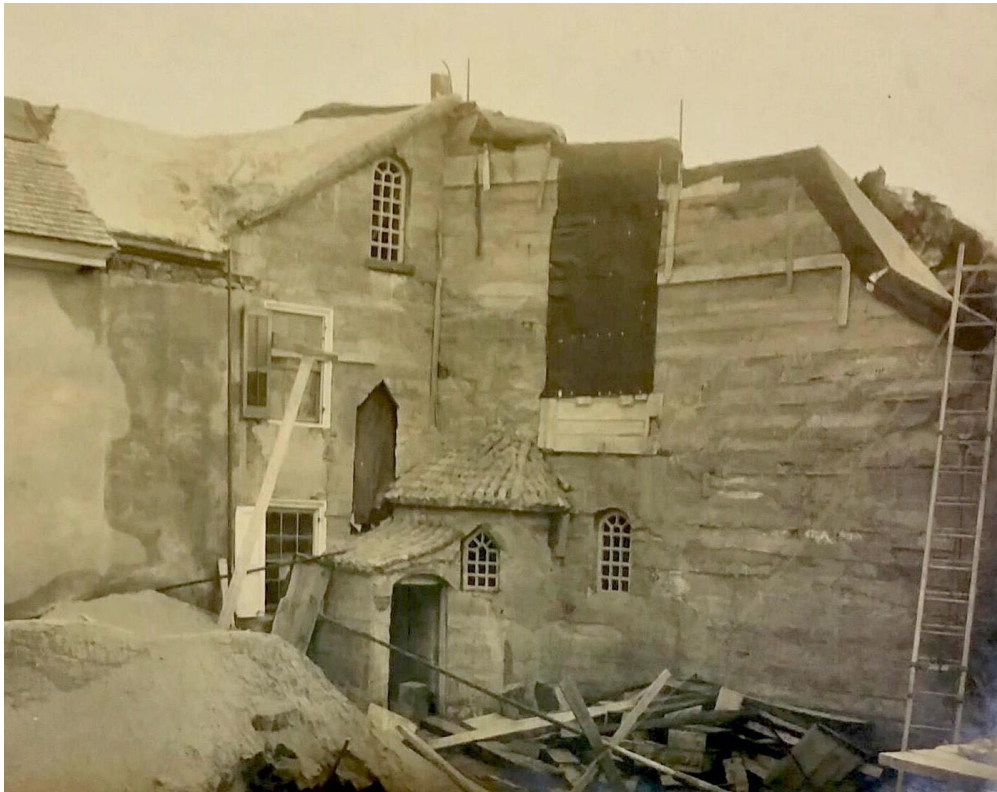
Figure 3.17. Rear facade of Fonthill, ca. 1908, with first story and part of second complete, showing what may be the first experiments in cast concrete windows. Image: courtesy of the Mercer Museum Research Library.
