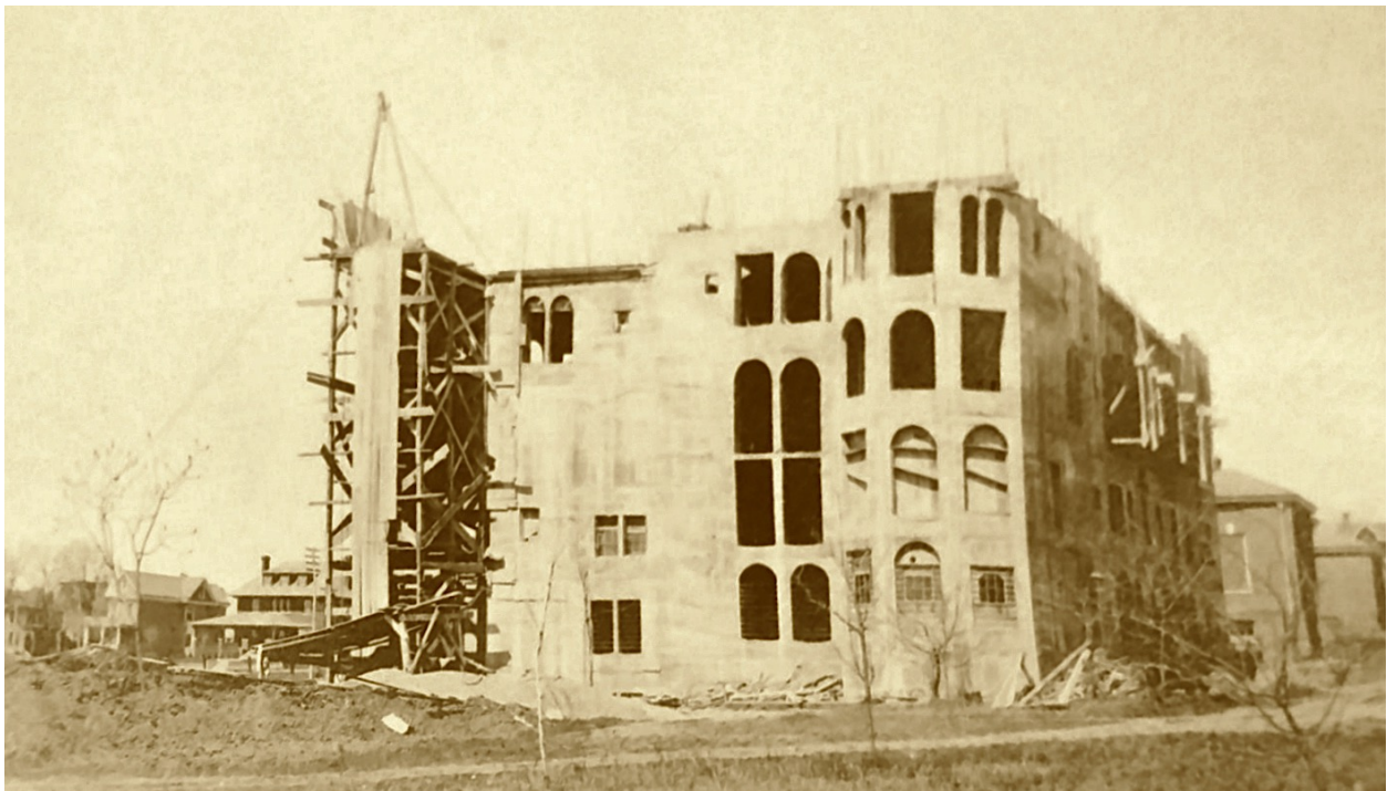
Figure 2.8. The museum, partially complete, with wooden crane to upper left. Note the faint lines of rebar extending vertically from the top level. Image courtesy of the Mercer Museum Research Library.
