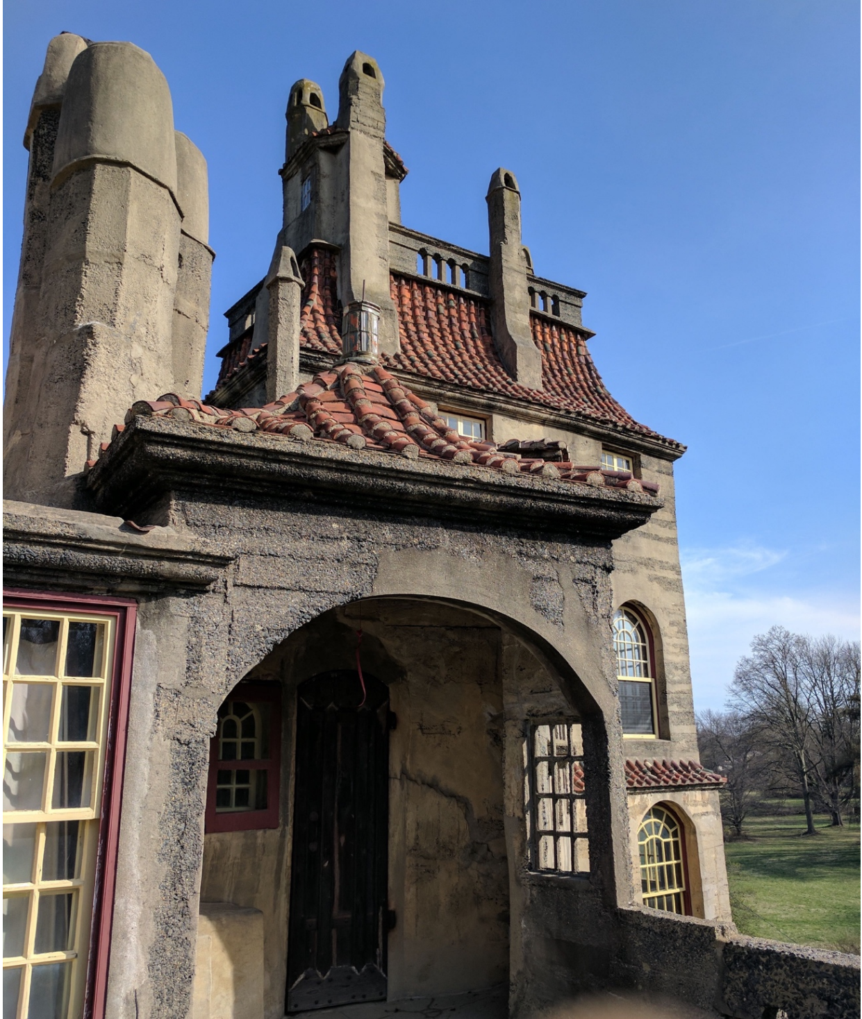
Figure 1.11. Exterior parging, Fonthill. Note the abrupt shift from unparged to parged surface half way through the arch in the foreground, and the complete reconstruction of the arched window opening in the right/background. These are areas that would be prone to initial failure (e.g., honeycombing) of the concrete work. Image: author.
