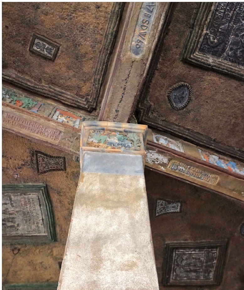
Figure 7.8. Saloon ceiling. Image: author, courtesy of Fonhill Castle.
