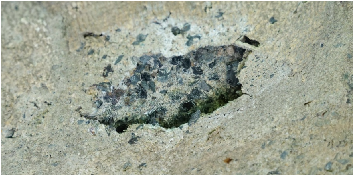
Figure 1.30. Failure at the cold joint between concrete layers, Moravian Pottery. We can conclude that this was a failure between cast-in-place layers rather than between concrete and parging because the surface layer retains the burlap texture characteristic of the exposed cast-in-place ceilings in this area, something that will be discussed later. Image: author.
