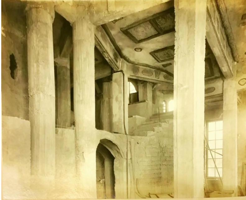
Figure 1.12. Interior prior to parging, Saloon room, first floor. Photograph taken during construction. Image: courtesy of the Mercer Museum Research Library.
