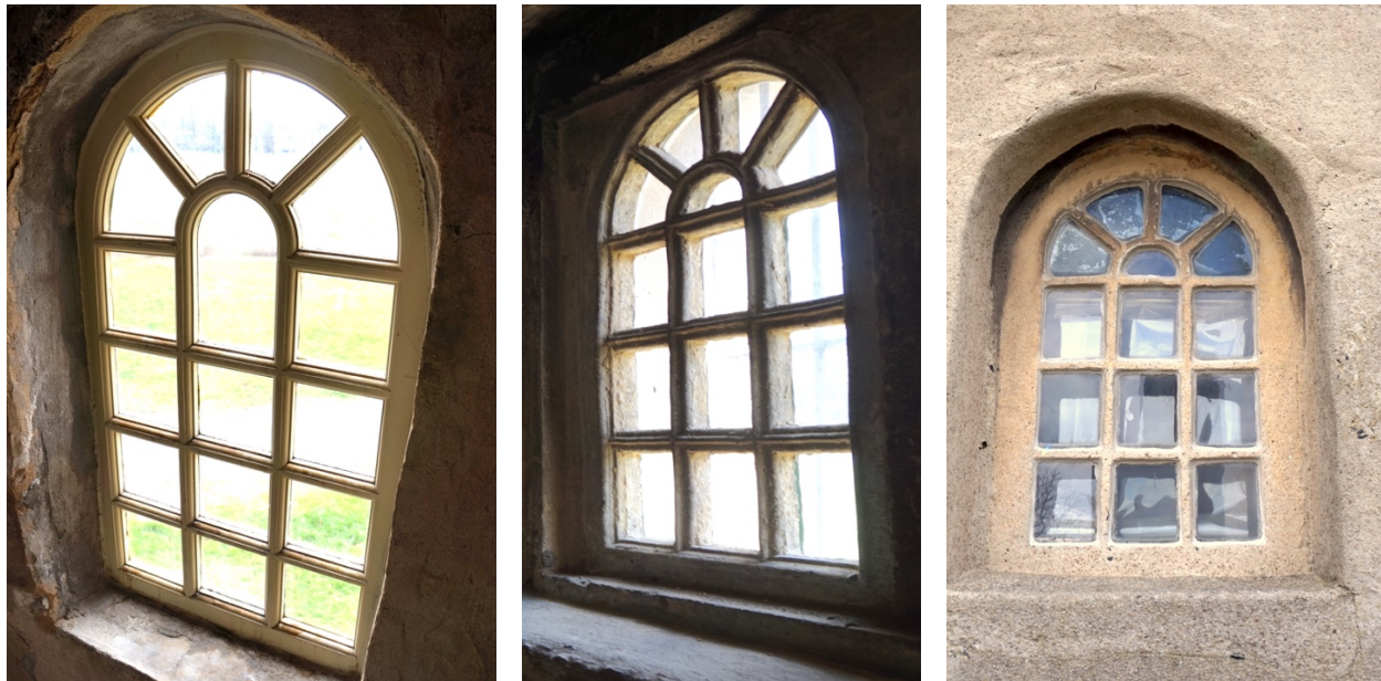
Figure 3.12, 3.13, 3.14. Wood and precast concrete windows, Fonthill. Images: author, courtesy of Fonthill Castle.
