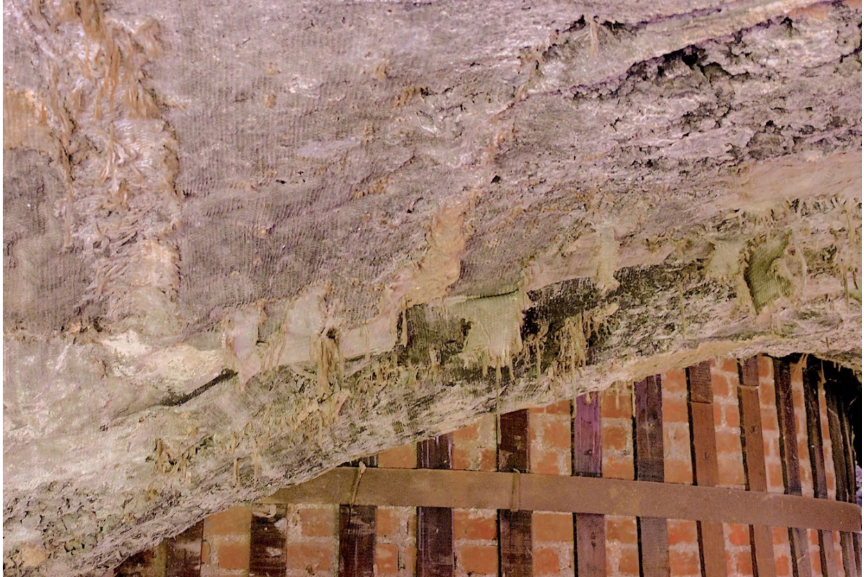
Figure 2.1. Carpet fragments adhered to concrete ceiling, with iron-band-reinforced brick kiln wall beyond. Moravian Pottery and Tileworks. Image: author, courtesy of the Moravian Pottery and Tileworks.
