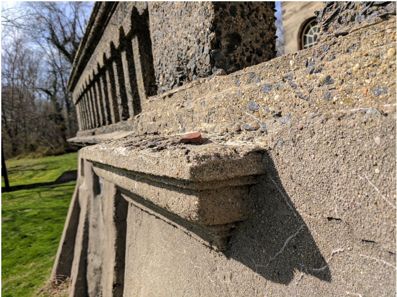
Figure 4.17. At Fonthill: cornice transitioning from wall surface, to flat roof condition. Image: author.
