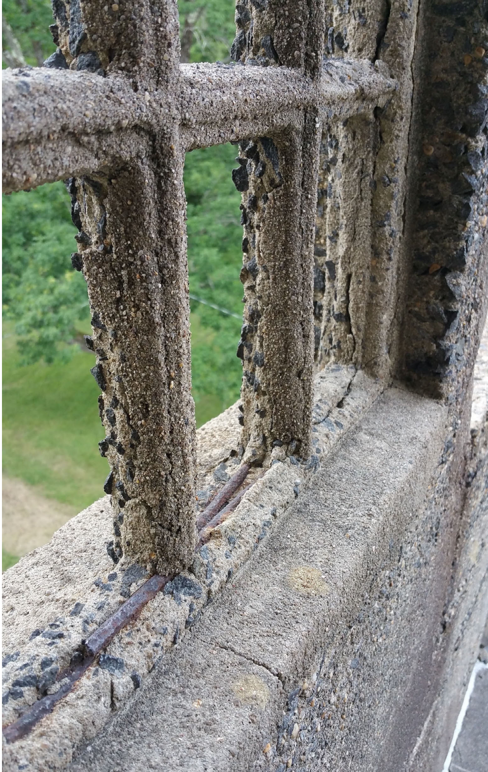
Figure 3.23. Muntin in unglazed window at outdoor terrace at Fonhill, showing corroded reinforcing. Freeze-thaw cycles may have exacerbated issues of insufficient coverage in this case. Image: author.
