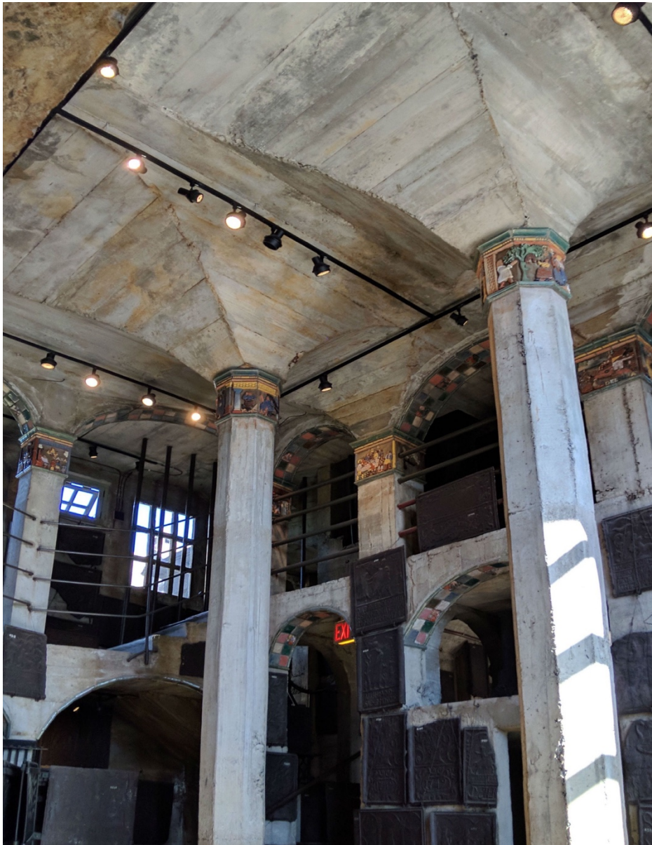
Figure 6.9. Boardform groin vaults in the stove plate room at the museum. Image: author, courtesy of the Mercer Museum.
