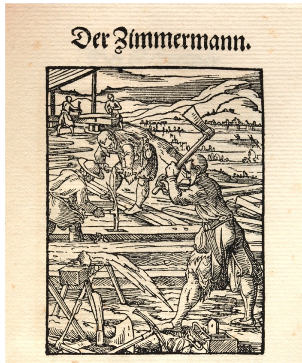
Figure 5.22. Use of the drawknife to plane timber. The carpenter in the foreground is at work with a medieval frame saw; the carpenter in the background is planing a beam or plank (the image is unclear) with a drawknife. Image: Der Schreiner. Hans Sachs, in Jost Amman’s 1568 Daily Description of all Occupations on Earth .... / public domain.
