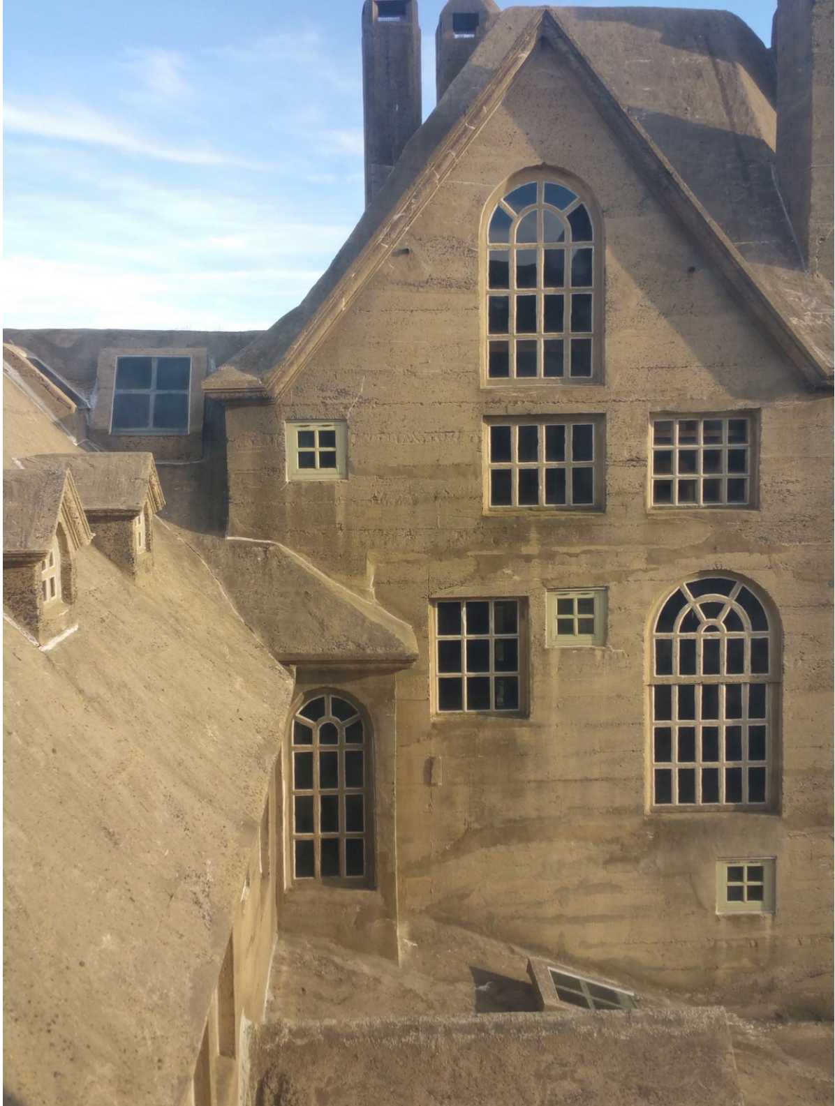
Figure 4.11. Cornice at the Mercer Museum. Image: author.
