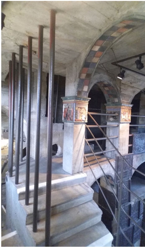
Figure 2.12. Pipe used as cast-in-place floor to ceiling balusters in the stove plate room balcony. Image: author, courtesy of the Mercer Museum.
