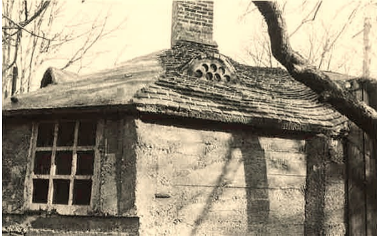
Figure 3.20. Eyebrow dormer and full window detail view. Archival image of Mercer's first experiments in concrete. Image: courtesy of the Mercer Museum Research Library. Collection on loan from the Moravian Pottery and Tile Works.
