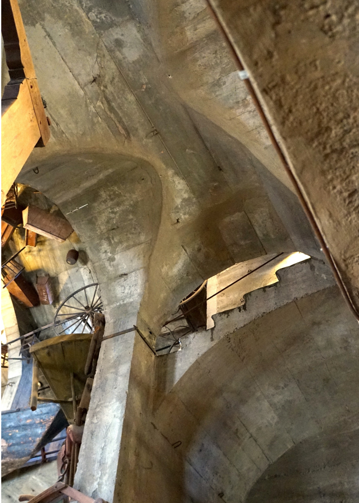
Figure 2.10. Museum, typical concrete vaults. Image: author, courtesy of the Mercer Museum.
