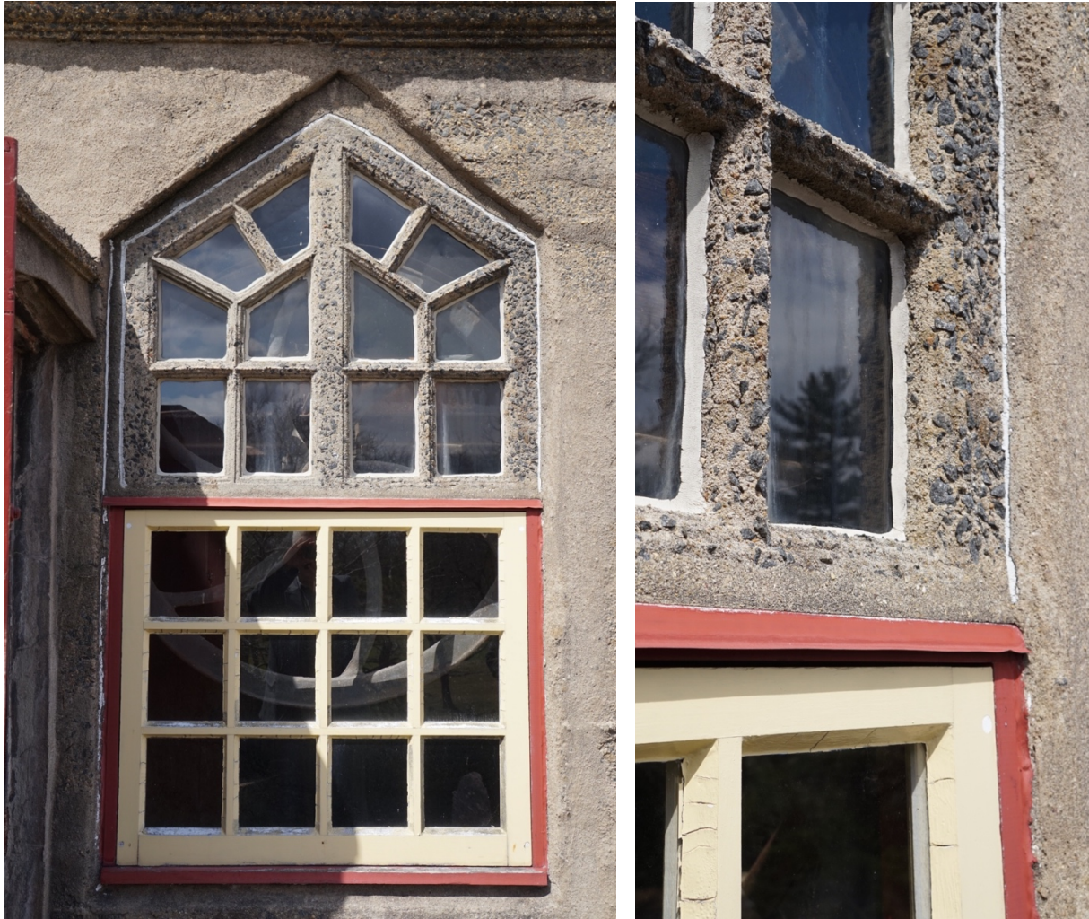
Figure 3.15, 3.16. Combination wood and concrete window at Fonhill. Note the ‘millwork’ profiles of the concrete muntins. In this case the upper concrete sash was installed ‘inside-out’, as the space behind it was an unfinished elevator shaft. (The lower sash may have been wood to facilitate its removal for summer ventilation.) Images: author, courtesy of Fonhill Castle.
