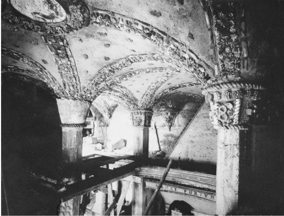
Figure 1.23. The library vaults under construction, after formwork removal and before column capital tiling was complete. Image: courtesy of the Mercer Museum Research Library.
