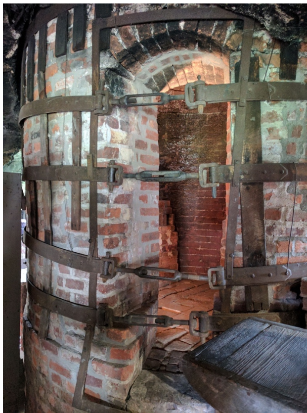
Figure 1.17. Bonts at one of Mercer's kiln openings. Image: author, courtesy of the Moravian Pottery.
