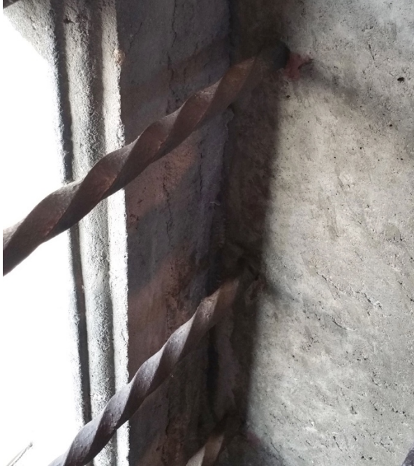
Figure 7.24. Twisted bar reinforcing passing through a window opening, finding economical use as a guardrail in Mercer's museum. Image: author, courtesy of the Mercer Museum.
