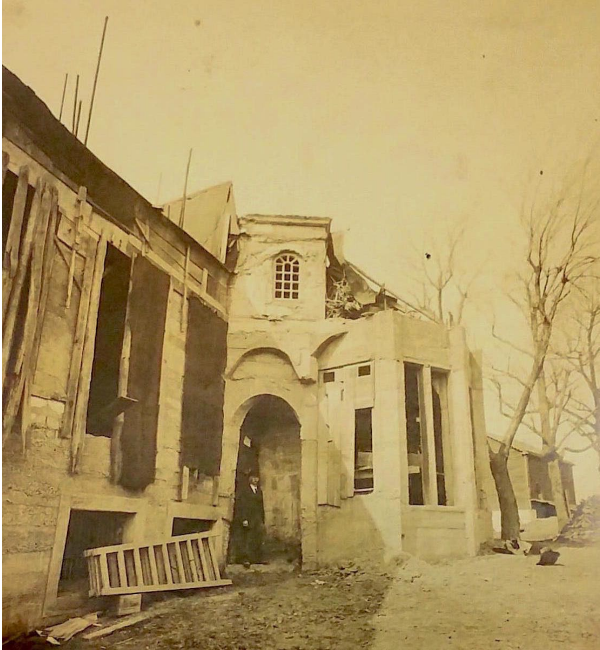
Figure 3.19. Front facade of Fontbill, ca. 1908, cellar and first story complete, showing what is likely the first wood window installed. Image: courtesy of the Mercer Museum Research Library.
