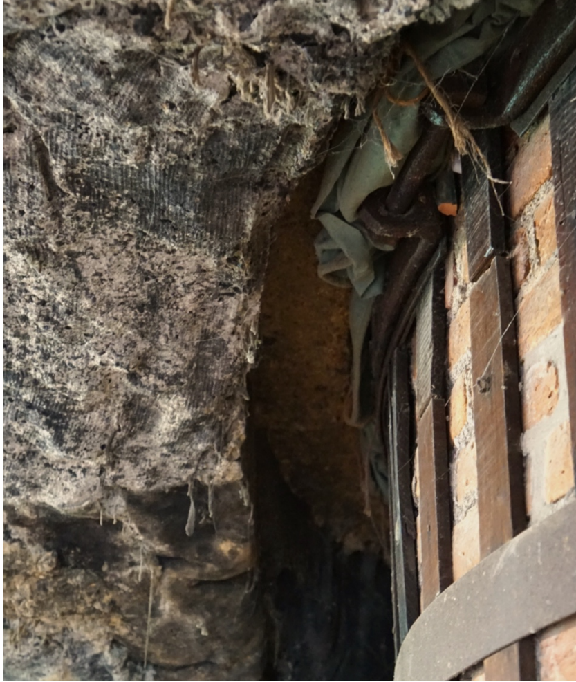
Figure 1.18. Gap between reinforced concrete vault and Bottle Kiln at the Moravian Pottery. This was likely intended to allow for thermal expansion during firing, and to avoid transferring load from the floor slab into the wall of the kiln. Kilns and Building were built separately, yet simultaneously. Image: author, courtesy of the Moravian Pottery.
