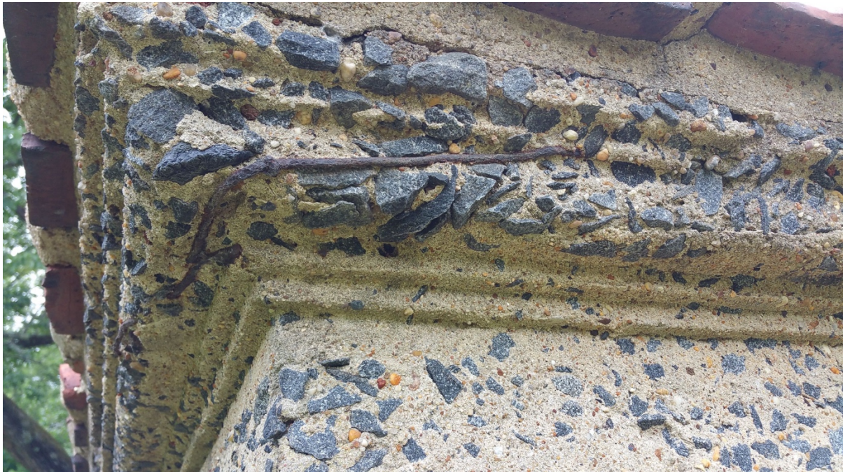
Figure 4.13. Cornice reinforcing visible at the spring house at Fonthill. Image: author.
