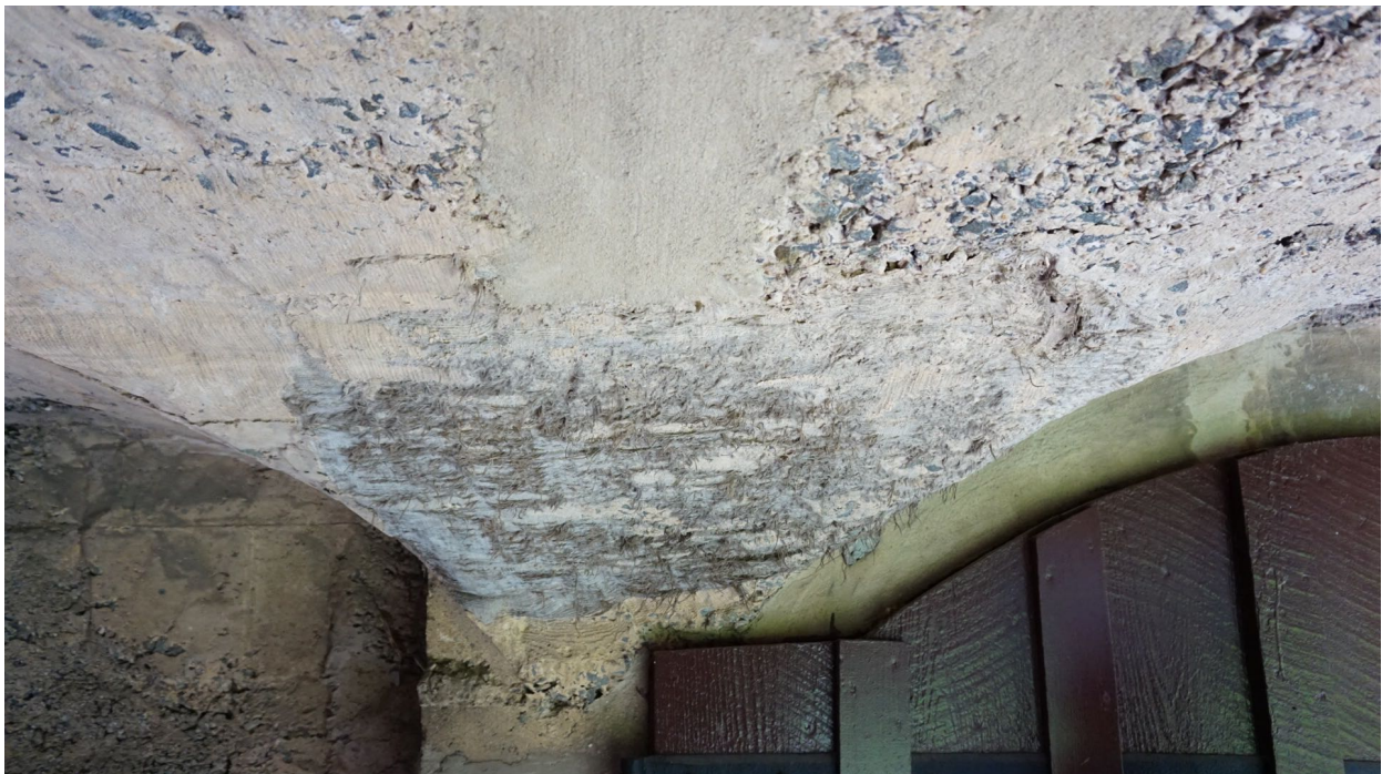
Figure 2.2. Burlap pattern in the cloister colonnade, Moravian Pottery. Image: author.
