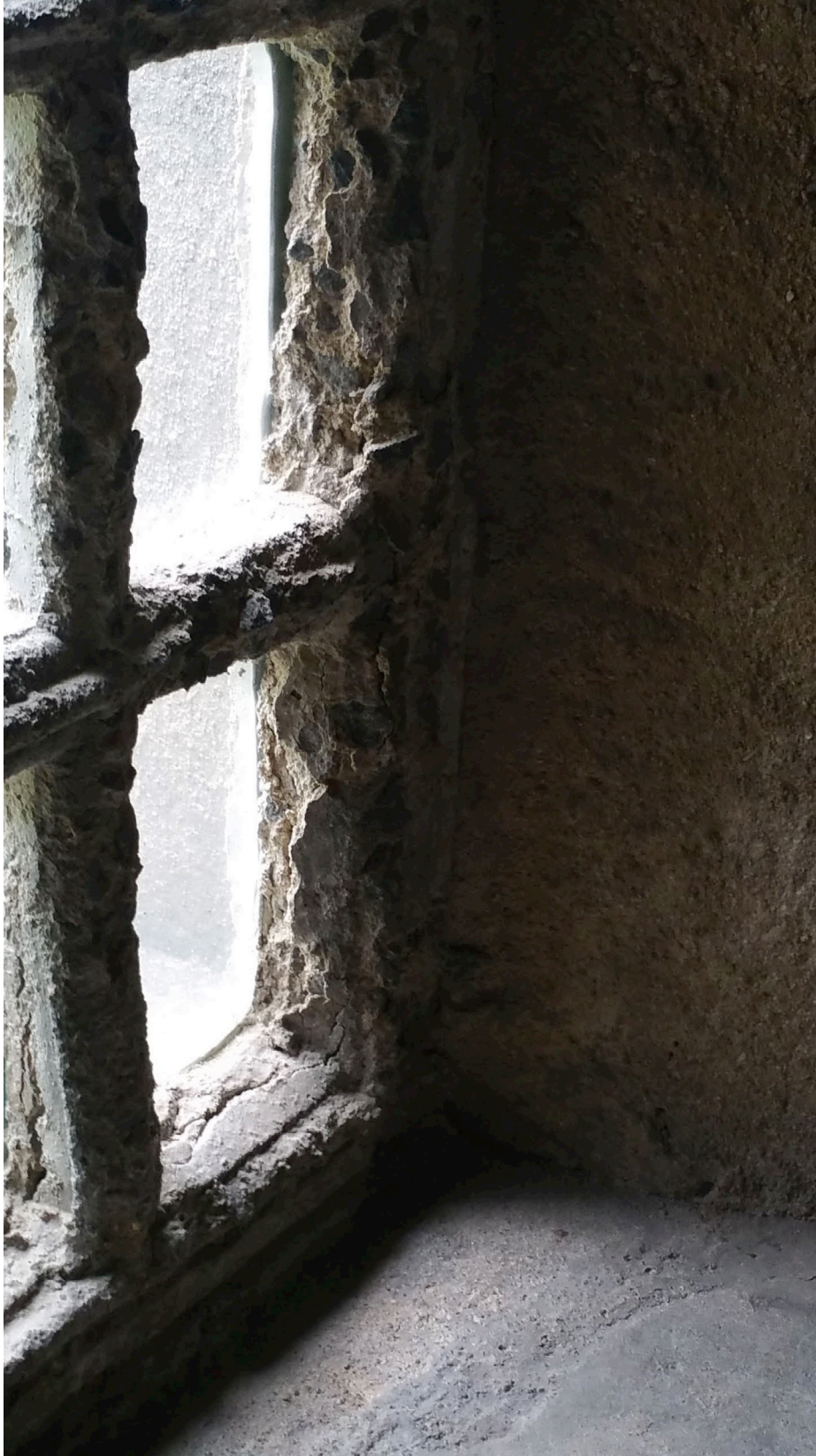
Figure 3.24. Degraded precast window with muntin profiles mostly effaced, Fonthill. Image: author.
