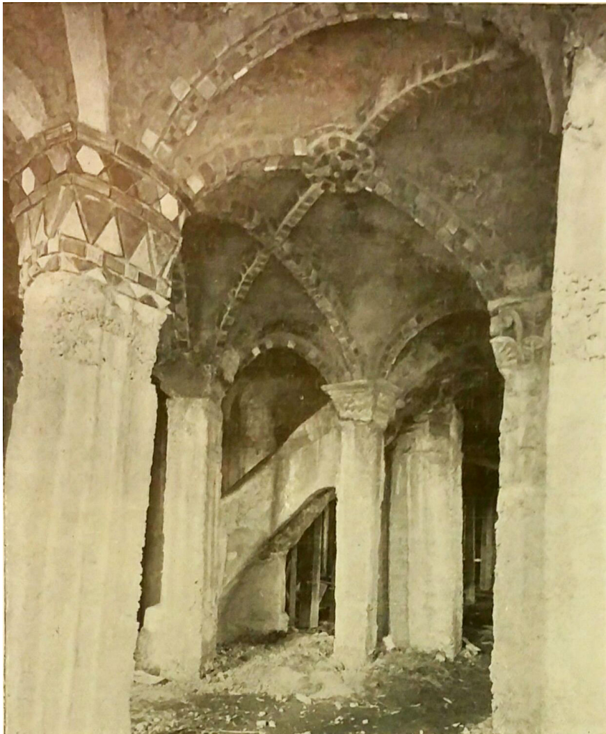
Figure 1.22. Construction photo, Fonthill, after formwork removal and before finishing. Image: "A Concrete House" Cement Age, May 1909 / public domain.
