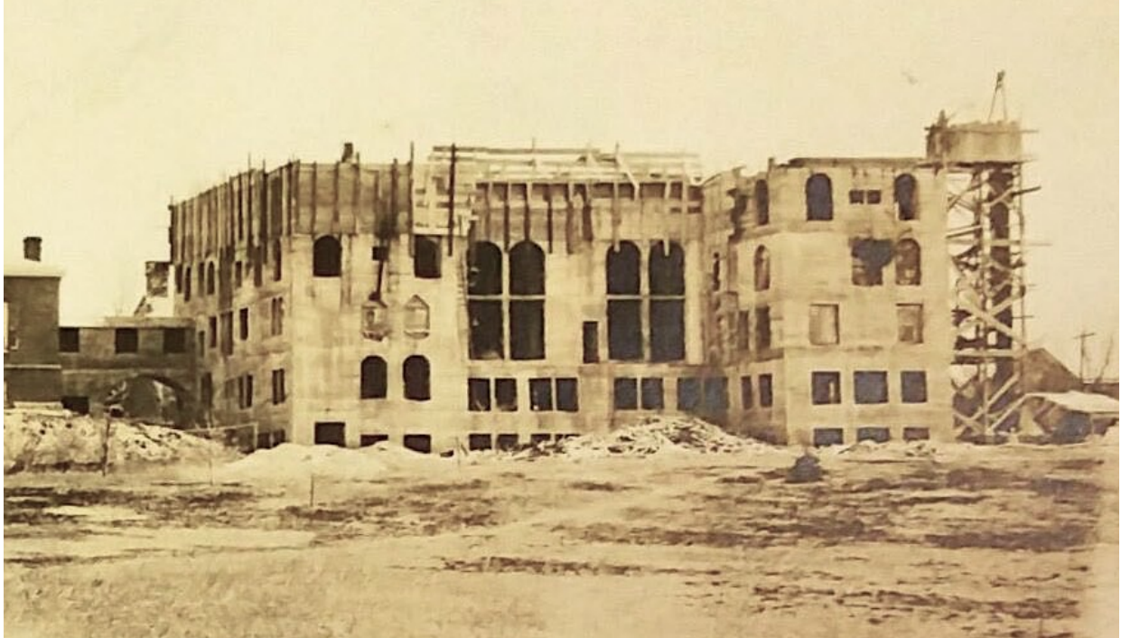
Figure 2.11. Formwork in place, and stripped formwork at the base of the museum under construction Image: courtesy of the Mercer Museum Research Library.
