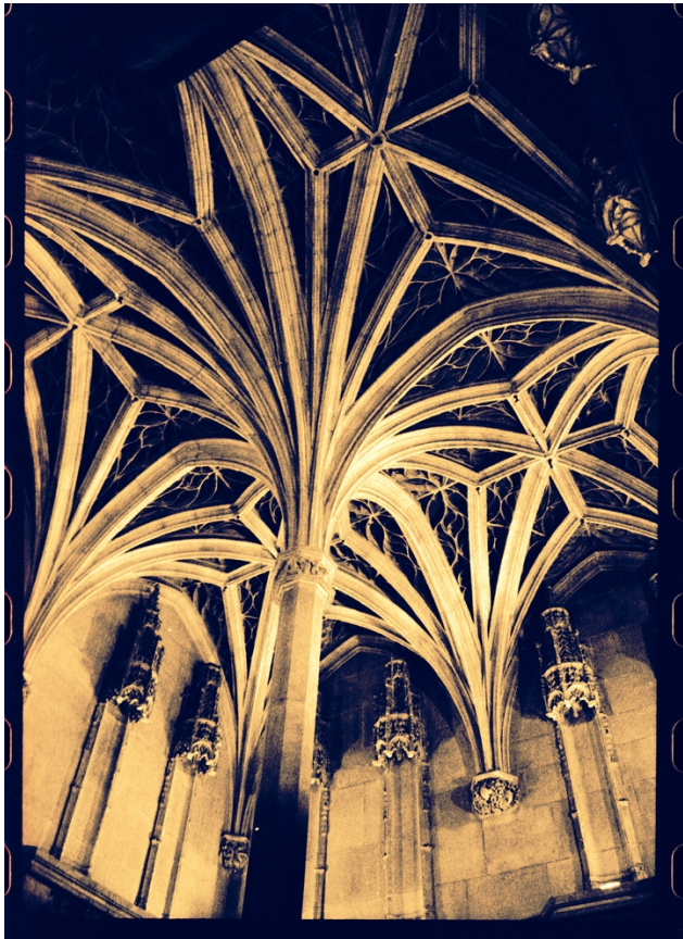
Figure 7.4. A chapel at Cluny, Paris. Note the placement of a single column in the center of the room, typical for a chapter house. Mercer may have been influenced by this particular idea, as many of his rooms feature a single, central, column. In the pottery, for example, the workspaces are configured as a series of rectangular rooms side-loaded along a colonnade, with a column roughly centered in each space. Image: author.
