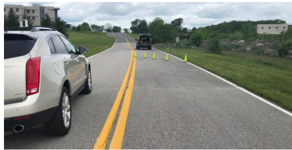
Figure 14: Lane shift location for work zone.
