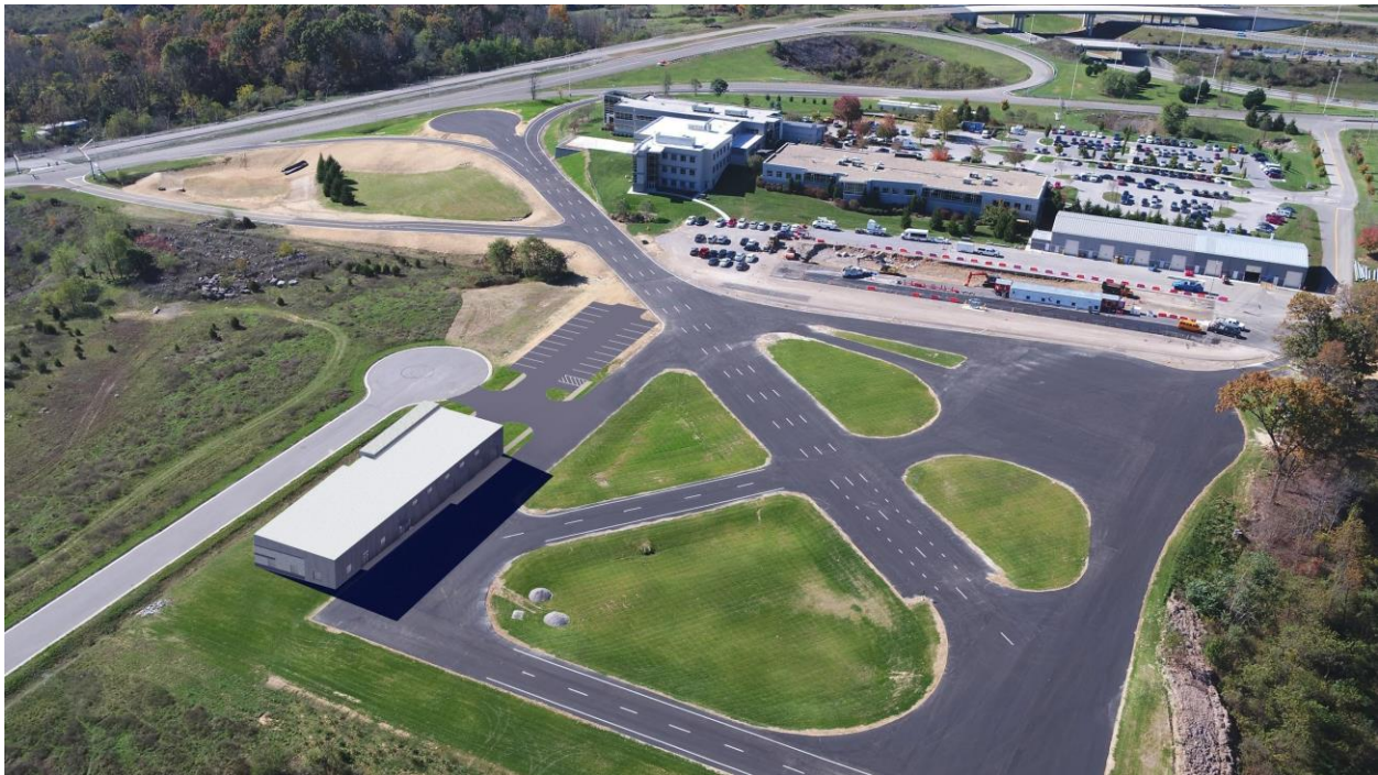
Figure 2: Top-down view of the Surface Street (foreground) and highway (background) sections of the Smart Roads used for testing.
