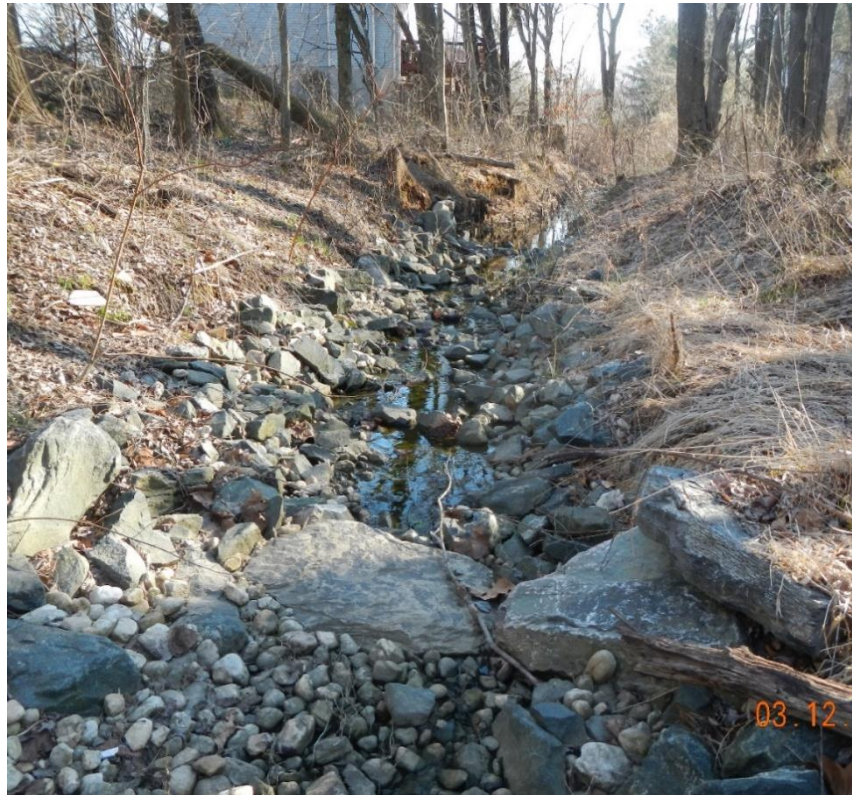
Figure 4-9 Representative photograph of project 47
