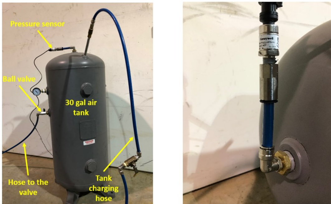
Figure 4.4: Multiport air tank (left); mounted pressure sensor (right)
