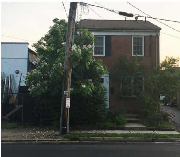
Figure 39. Conflict in Transitional Edge. The edge between this detached residence on the Wythe Block and the adjacent loading dock/fenced storage area of Alexandria Lighting & Supply (pictured to the left) shows evidence of conflict. Note the abundance of residential plant material used to obscure the edge.
