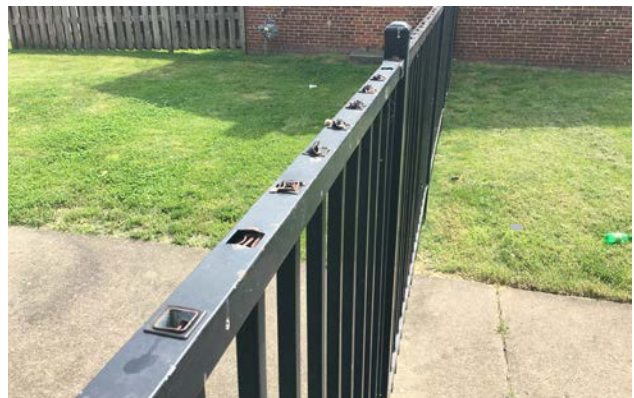
Figure 33. Spiked Fence Tops Removed, Samuel Madden. At some point after installation, the spiked fence tops appear to have been pried off of the six-foot fence at Samuel Madden.
