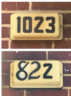
Figure 35. Porch Lights, Samuel Madden. Back-lit house numbers function as porch lights on the garden-style units at Samuel Madden. Some lights (bottom) have been repaired in ways that add even more vernacular character.
