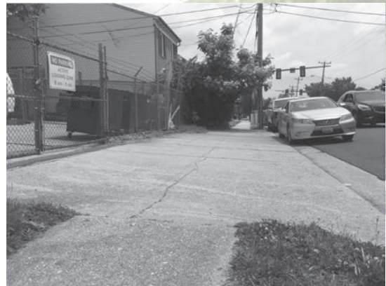
Only 16 feet of the 48-foot loading dock are used for loading; the balance is defined by an inactive impermeable boundary fence. This image looks east past the loading dock and fenced storage area toward the arbor.
