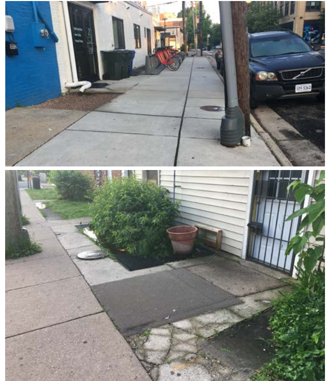
Figure 34. Social Edge Revealed through Infrastructure. The social edge marking the transition between existing and gentrified businesses on the south side of the Madison Block is revealed in the character of the adjacent sidewalk. A freshly paved and scored sidewalk (top) serves the newly redeveloped buildings, while the sidewalk adjacent to the existing Community Market and barber shop (bottom) is a collection of makeshift concrete patches signifying a pursuit of accessibility around the City’s utility poles.
