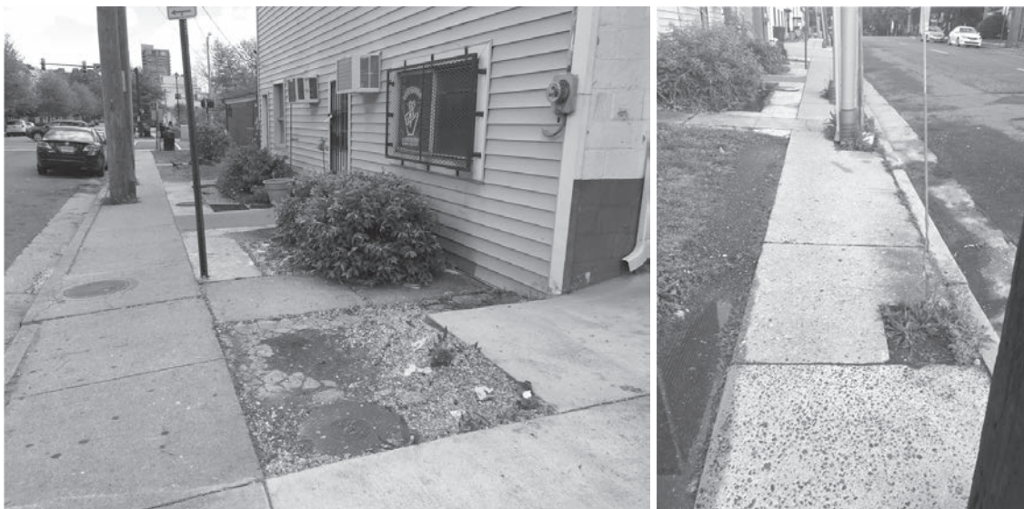
Accessibility and maintenance issues are observed adjacent to the Community Market and barber shop (background). Note the utility poles and signage blocking the pedestrian zone and the makeshift concrete patches that have been installed to maintain adequate width. The photograph on the left looks east, while the photograph to the right looks west.
