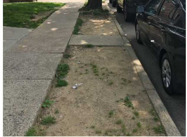
Figure 38. Compacted Soil in Continuous Tree Strip. Much of the soil within the continuous tree strip on the north side of the Madison Block is severely compacted, possibly by residents accessing parked cars or by residents engaged in staying.
