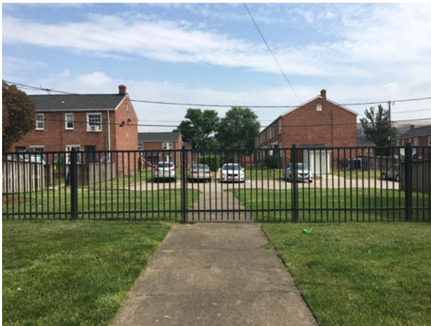
Figure 21. Public Housing Fencing. Black, powder-coated aluminum fencing is observed as a permeable border in three-foot, intermittent segments at Andrew Adkins (left) and as an impermeable boundary in a 6-foot gateless segment at Samuel Madden (top).
