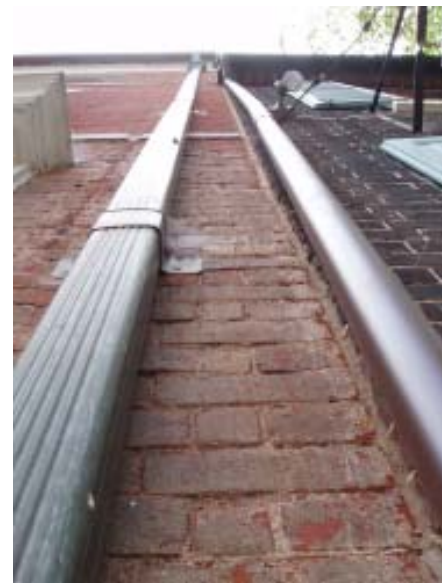
rain falls on rooftops and is drained through the rain gutters on a building
