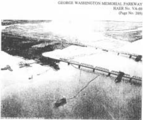
Figure 93 Dredge pumping (H) for Columbia Basin from bed of Potomac River, south of R&P railroad bridge, 1930 (Lee, "Final Report for the Construction of the Mount Vernon Memorial Highway")
