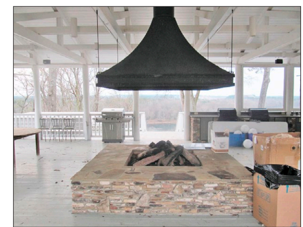
Suspended smoke hood for pavilion fire pit
