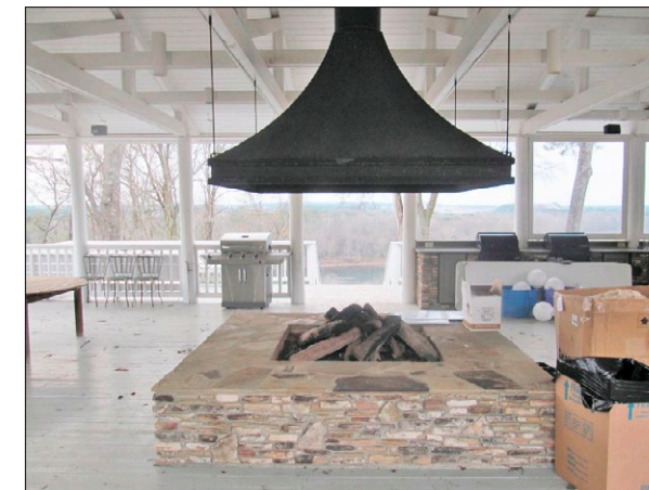
Suspended smoke hood for pavilion fire pit.
