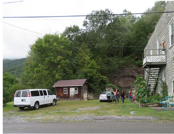
Parking, old shed, and exterior staircase for tenant entrance.
