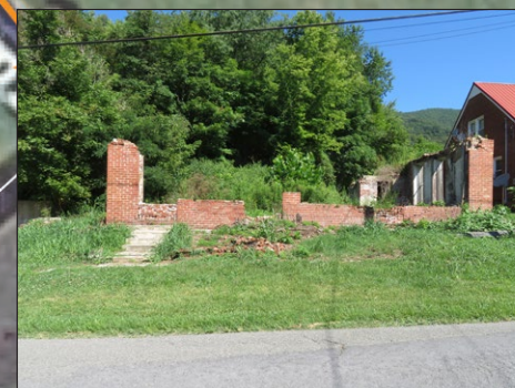
E. Front facade view of old bank building. Consider visual aesthetic for surrounding neighbors and photo opportunities for visitors.
