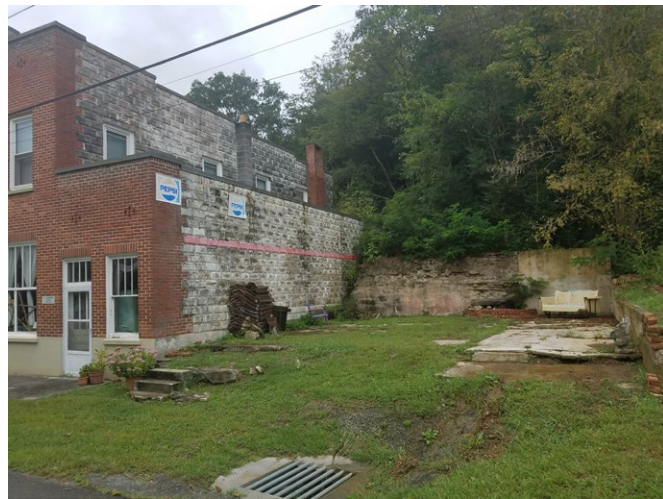
View into vacant lot adjacent to store building. During heavy rainfall, water runs from steep slope behind the bank building, under the concrete, and into the drain.
