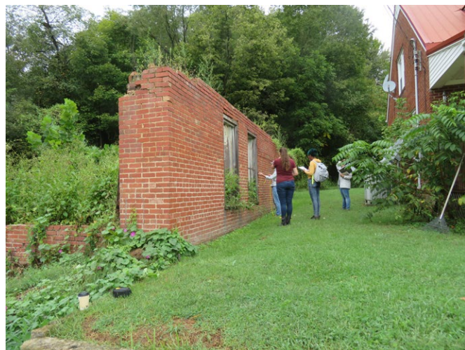
Northeast facade of bank building in close proximity to neighboring residence
