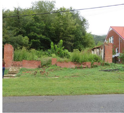
Remnants of former bank building with overgrown vegetation
