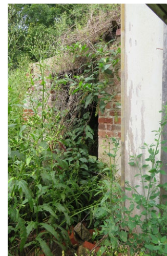
Existing bank vault to be incorporated into proposed design
