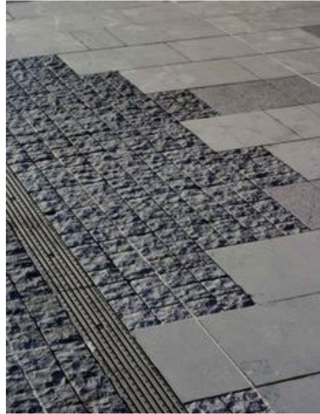
Paving Material Transition
