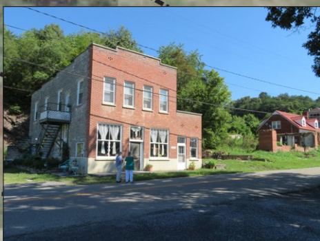
C. View from trailhead entry to general store and old bank building. Consider pedestrian connections when crossing Mendota Rd. and facade view that would attract visitors.
