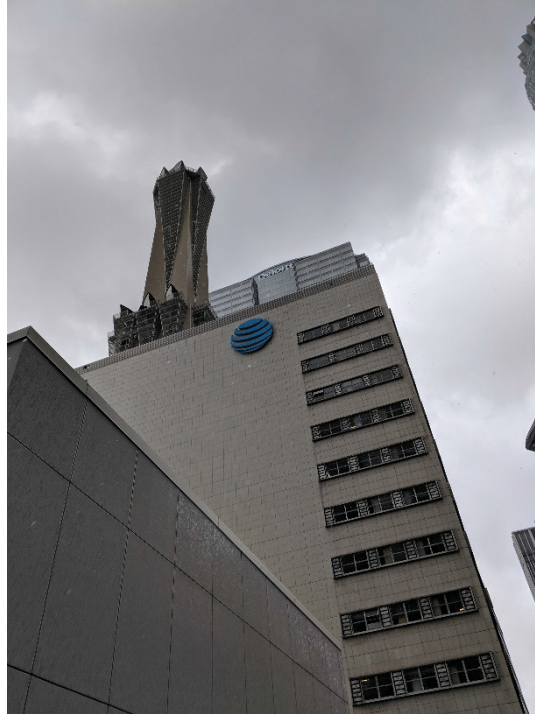
92. AT&T Switching Center (source: Trevor Croker)
