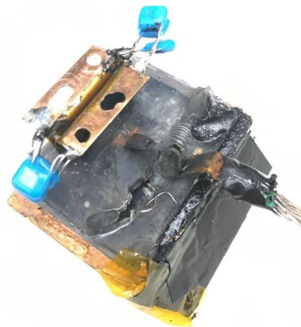
Figure 5-31. Module 6 after experiencing thermal runaway after 2-3 minutes at 250 V, 47.7 A input, 500 V, 23.86 A output
