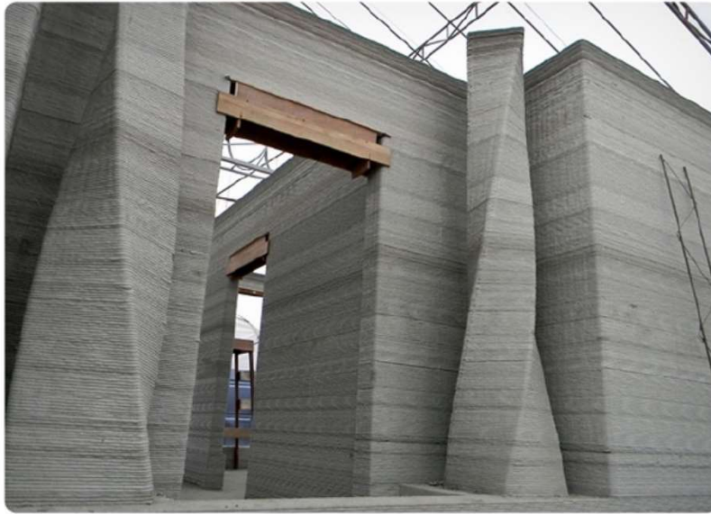
f) vertically printed, in-situ walls and columns. Image: courtesy of Andrey Rudenko, Total Kustom, USA
