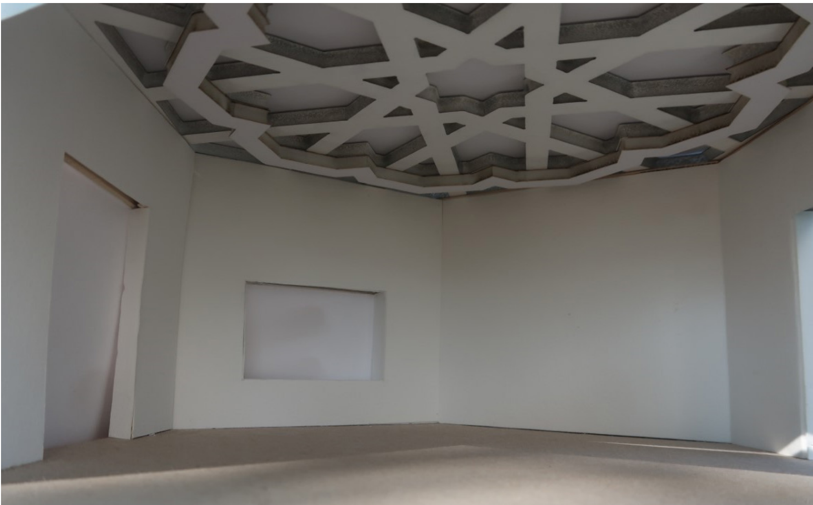
model study: interior view medium level activity class interior view.
