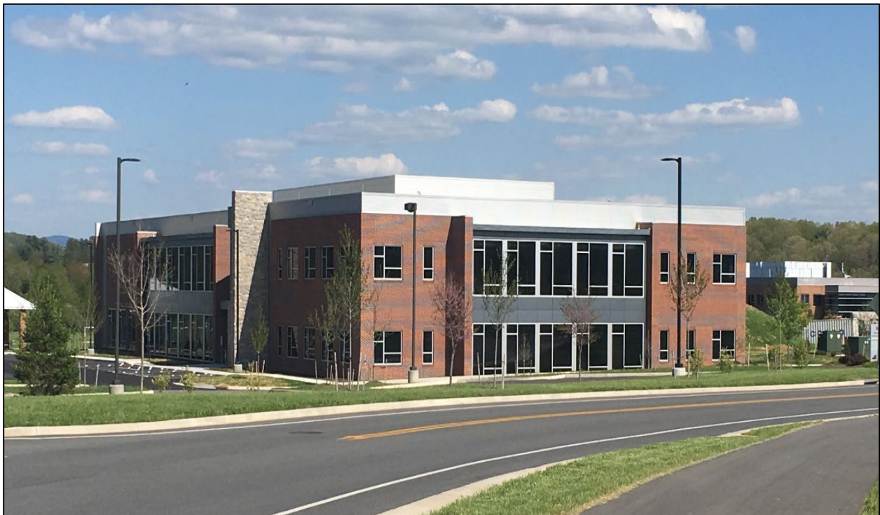
Figure 2: Photo of VTCRC 1311: Northwest Corner View (Stutesman, 2019)
